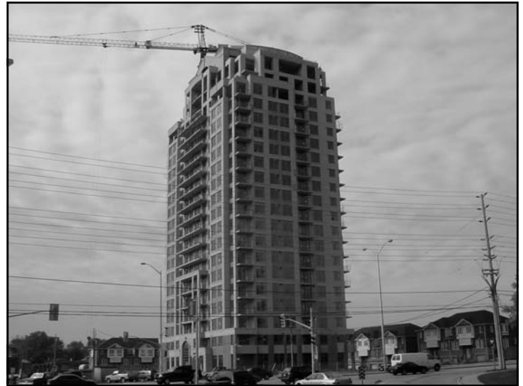
"The Capri" under construction in Rathwood
