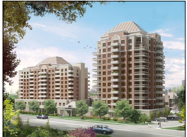
Development under construction at Eglinton Avenue and Mavis Road. Apartments such as these represent the source of much of the City's future housing starts with the end of greenfield development.
