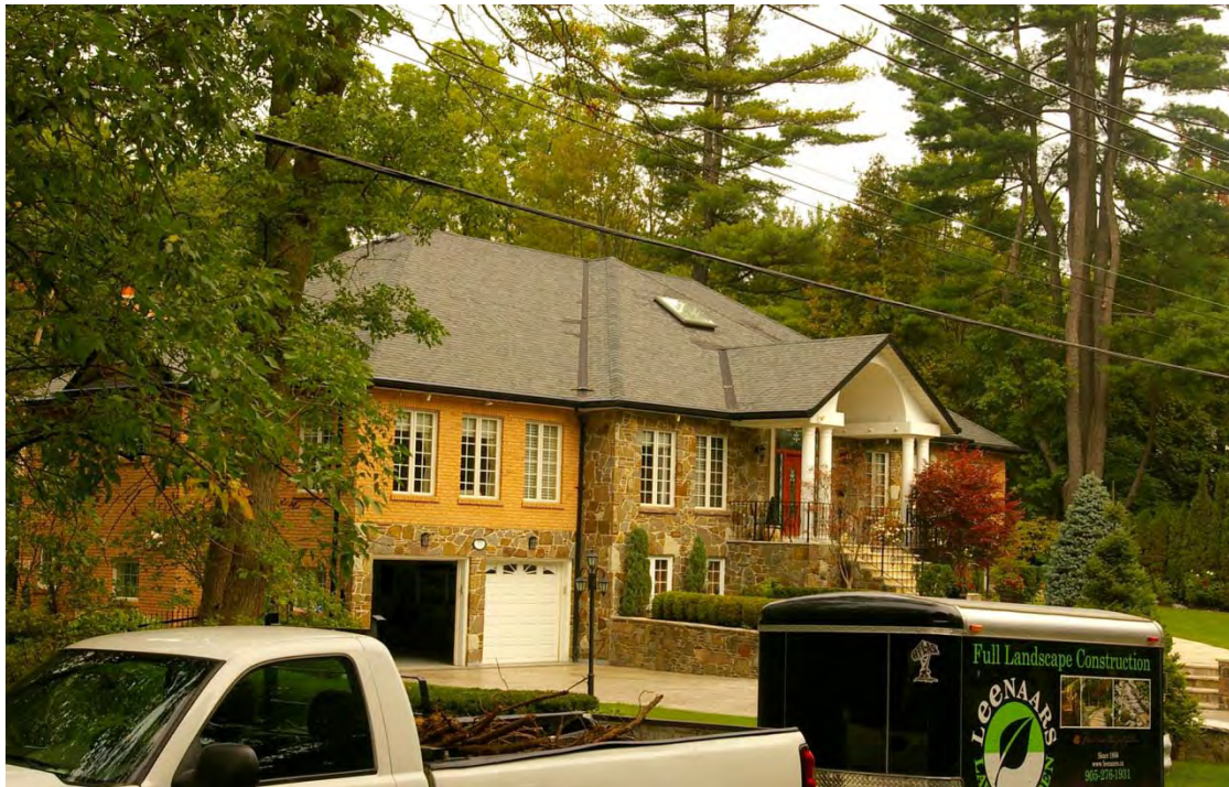
Photo 10: A replacement dwelling at 313 Indian Valley Trail, first built in 1993 but since renovated and enlarged. This raised bungalow with a two-car garage in the basement level is clad in brick and stone veneer. The driveway is surfaced with concrete.
