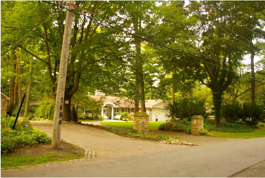
Photo 20: View of the house at 1448 Stavebank Road, which appears to be an original bungalow with an added portico and double garage.
