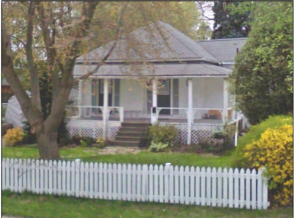
“Wrap-around” front porch, typical of earlier homes on John Street South.
