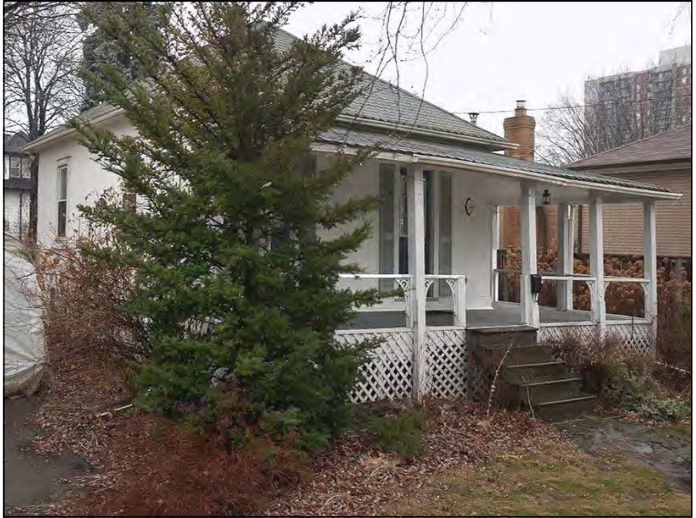
Front of main residence, looking west
