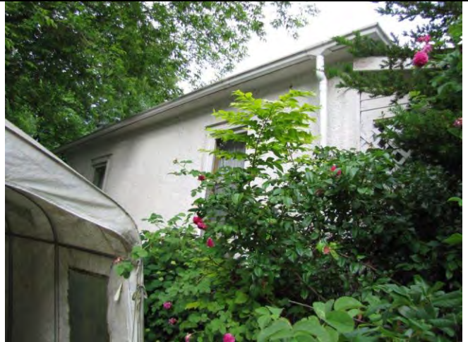
Photo 4: Side View Exterior
