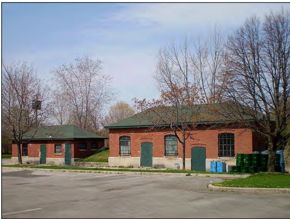
The Port Credit Public Utilities waterworks system began operation in 1923.
