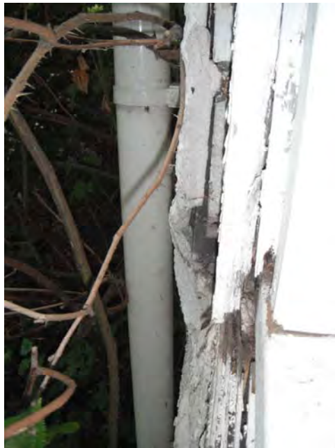
Stucco over wood trim
