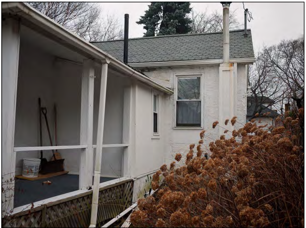
Corner of east-west and north-south axes of 24 John Street South.
