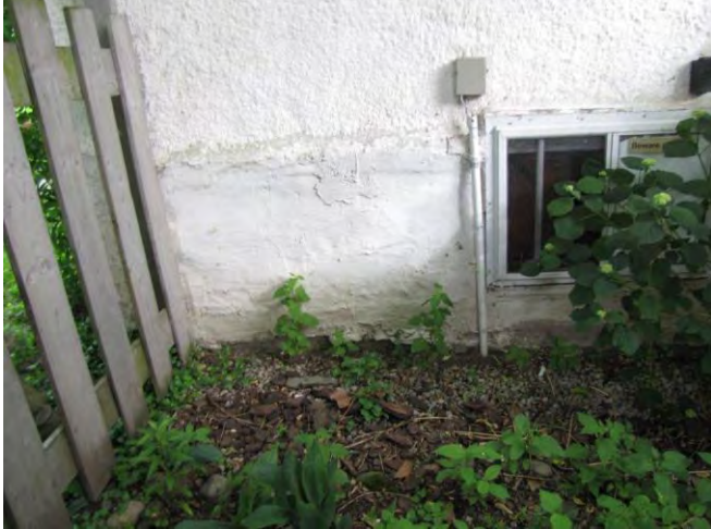
Parging repairs to the foundation.
