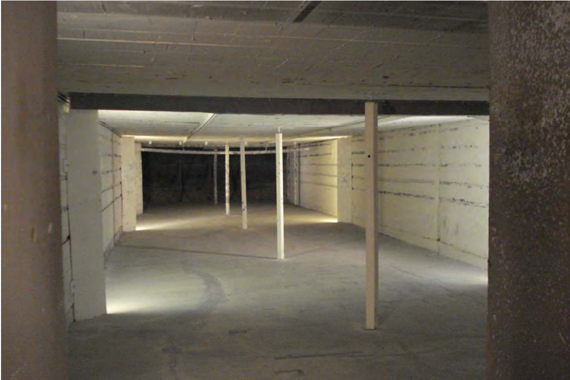
Interior facing Southwest
