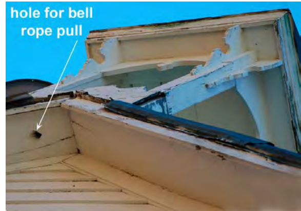
Figure 25 bell tower with bell rope pull hole
