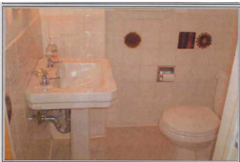
Fig. 27 Ground-floor Bathroom (powder room)
