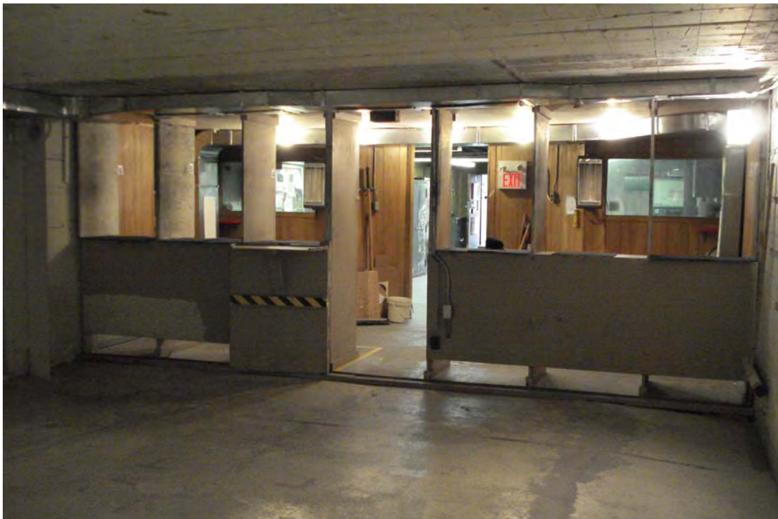
Interior facing Northwest
