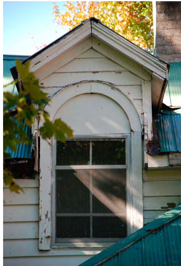
Figure 27 window head blocked-in with plywood
