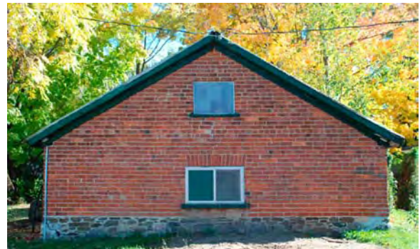
Figure 31 north elevation - dairy
