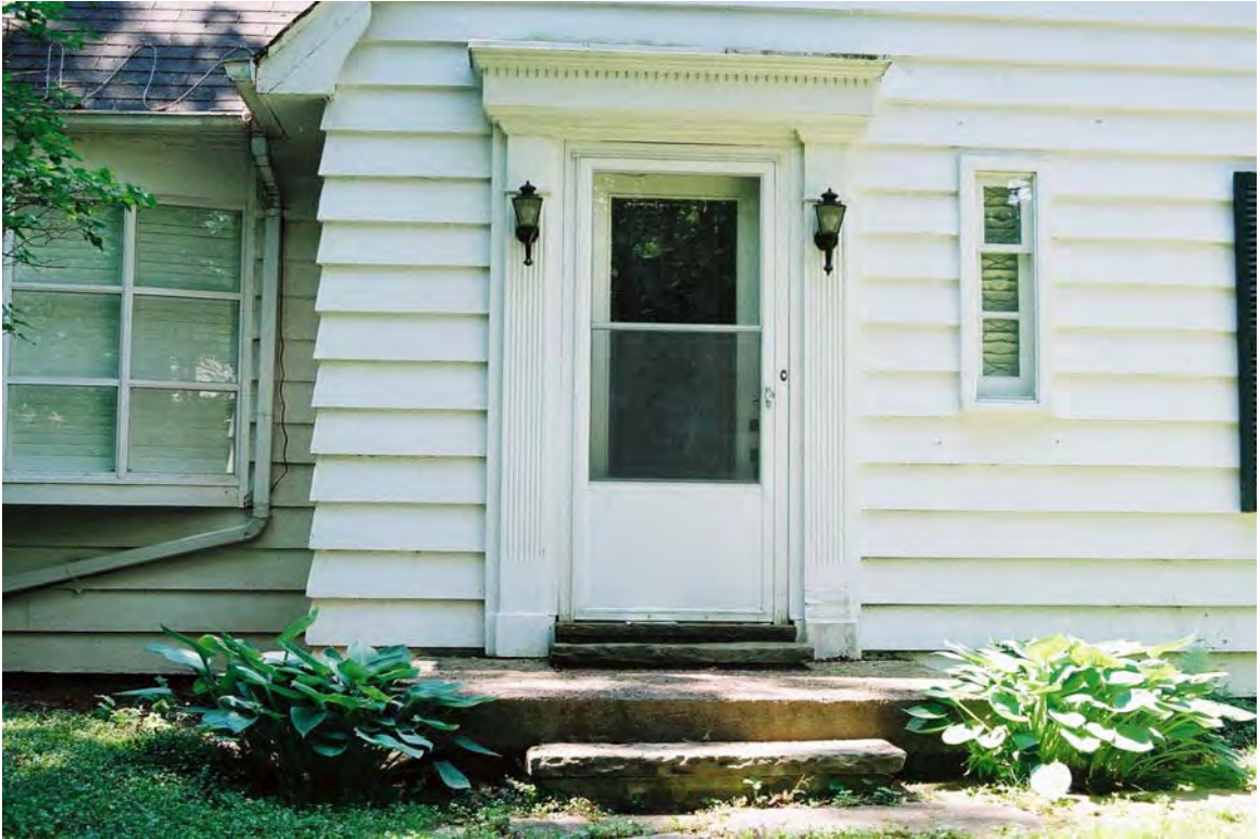
Fig. 19 Wide clapboard, Classical front entrance and Art Deco-inspired hall light
