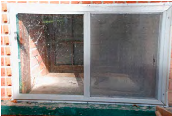
Figure 32 deep set window - dairy
