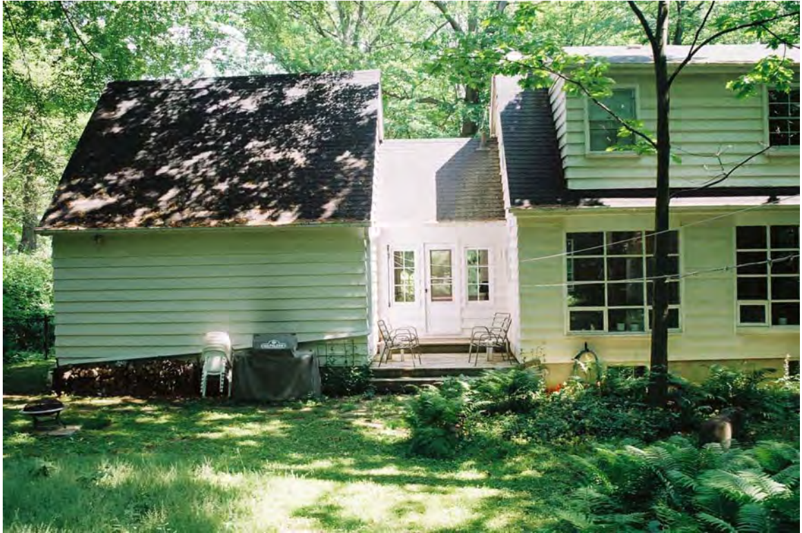
Fig. 21 Rear elevation of the garage, the interconnecting passage and a corner of the main house
