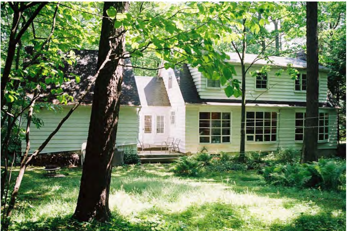
Fig. 20 House's rear elevation
