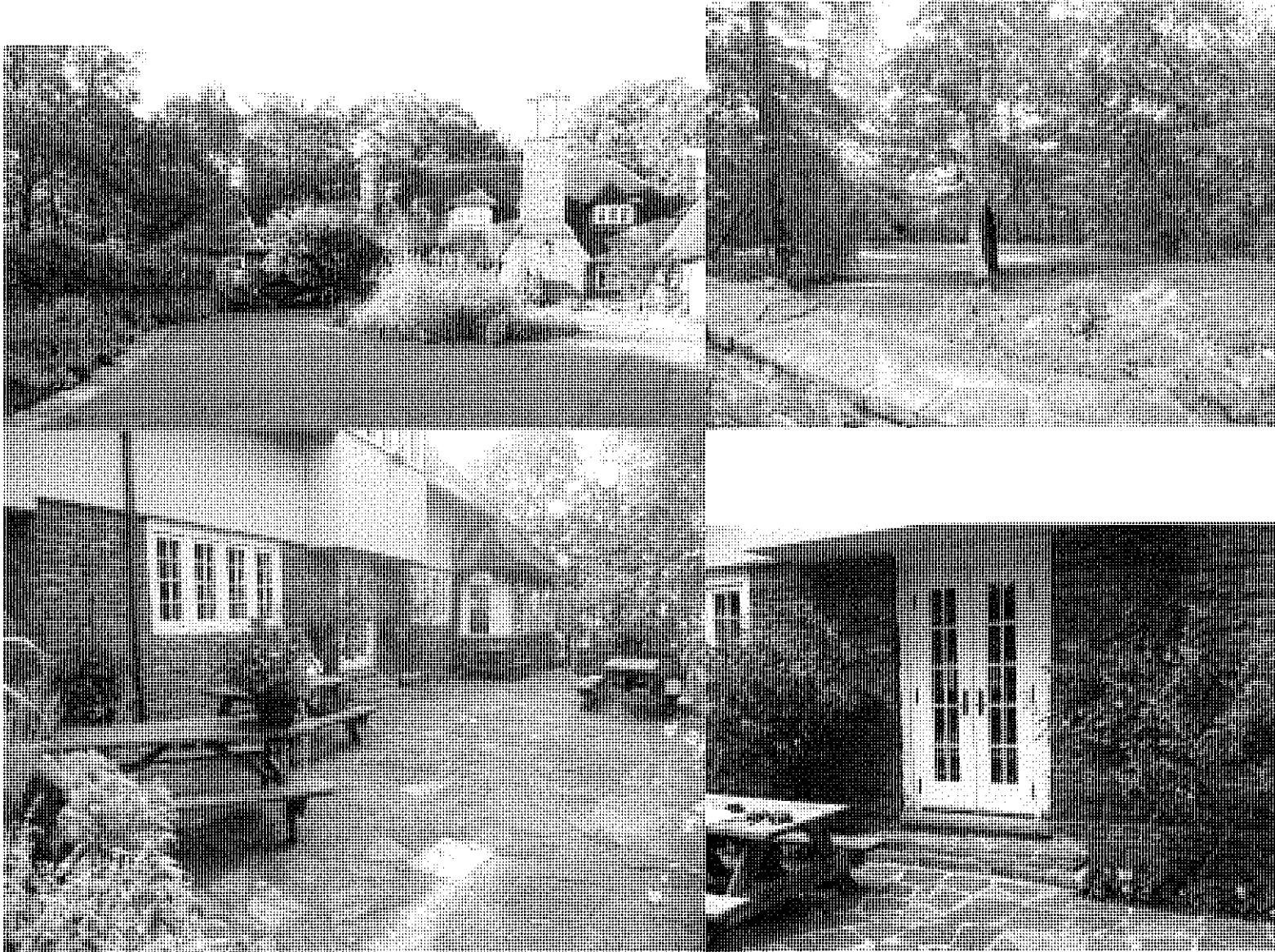
CHAPPELL ESTATE – EXISTING CONDITIONS 4300 Riverwood Park Lane September 2011
