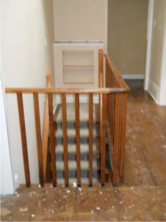
The upstairs hallway.
