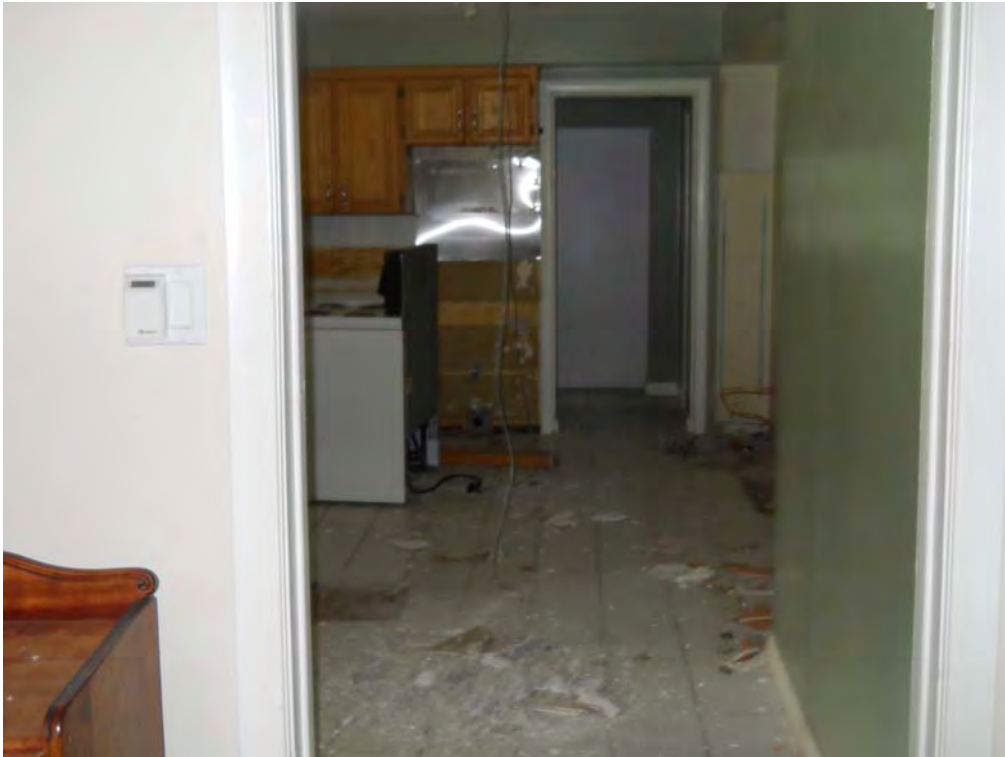
The kitchen; all fixtures have been removed.
