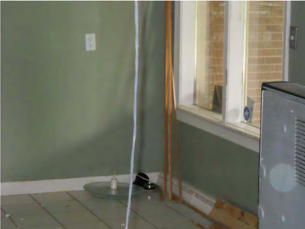
The kitchen; all fixtures have been removed.
