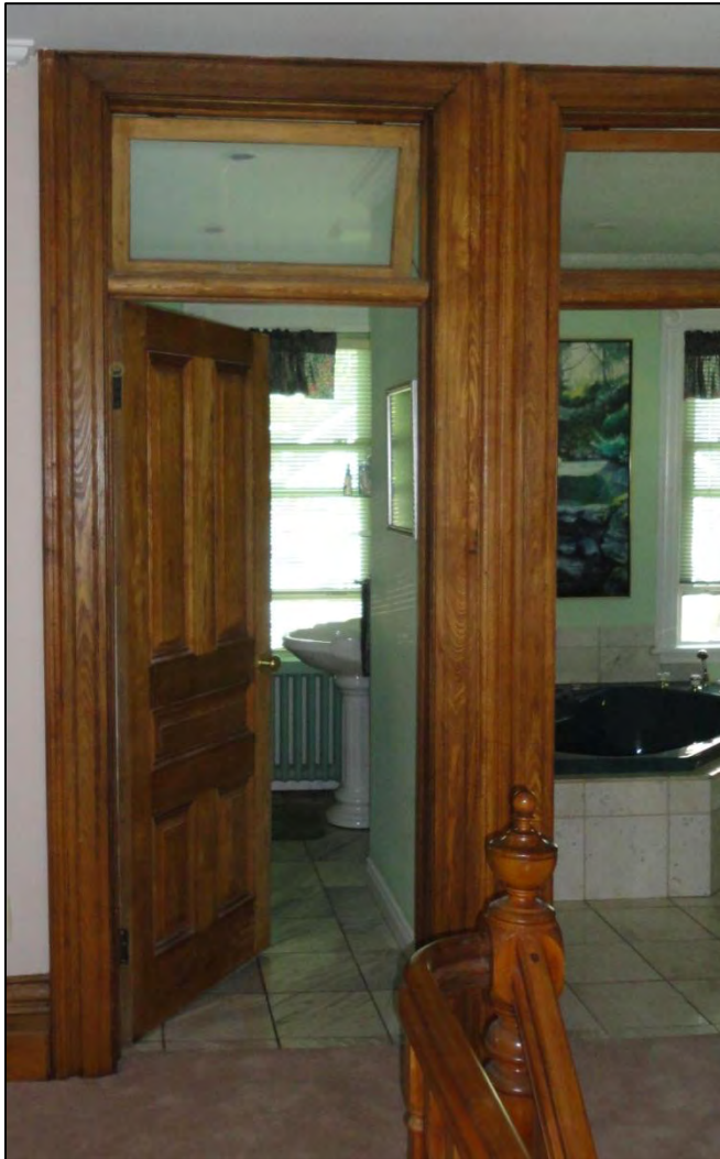
Upper Floor –Paired Room Entrances showing doors, casings and transoms
