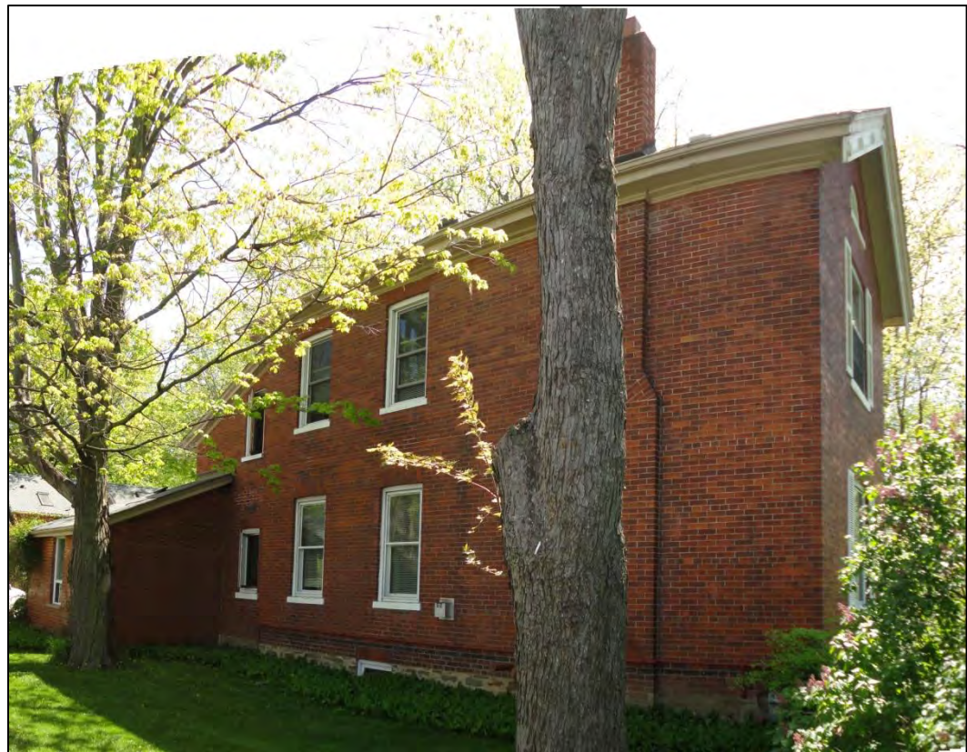
North Elevation, west end
