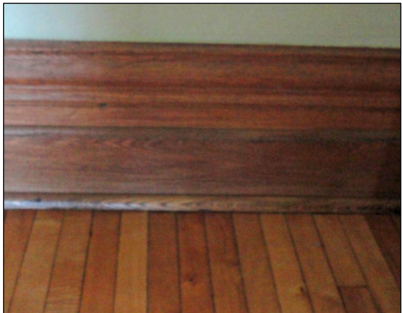
Ground Floor – North-west Room – baseboard and flooring detail
