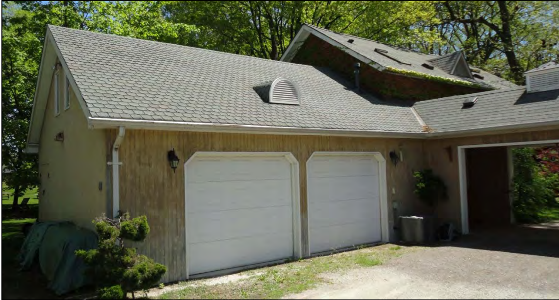
North and West Elevations, including garage addition
