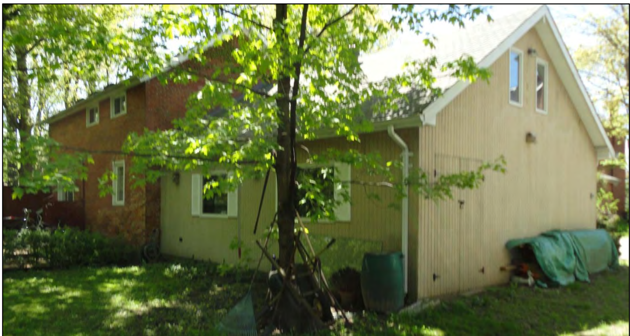
East and North Elevations including garage addition
