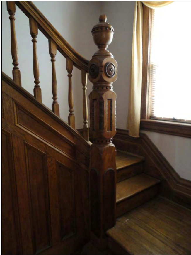
Ground Floor – Staircase – Newel Post, Balustrade and Box Panelling
