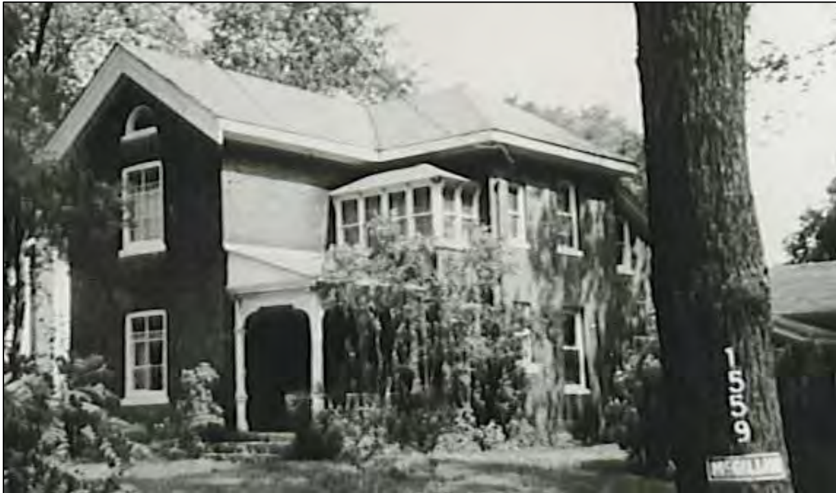
West and South Elevations, c. 1990 Source: Weeks/Mississauga Heritage Foundation/Helen McGillion
