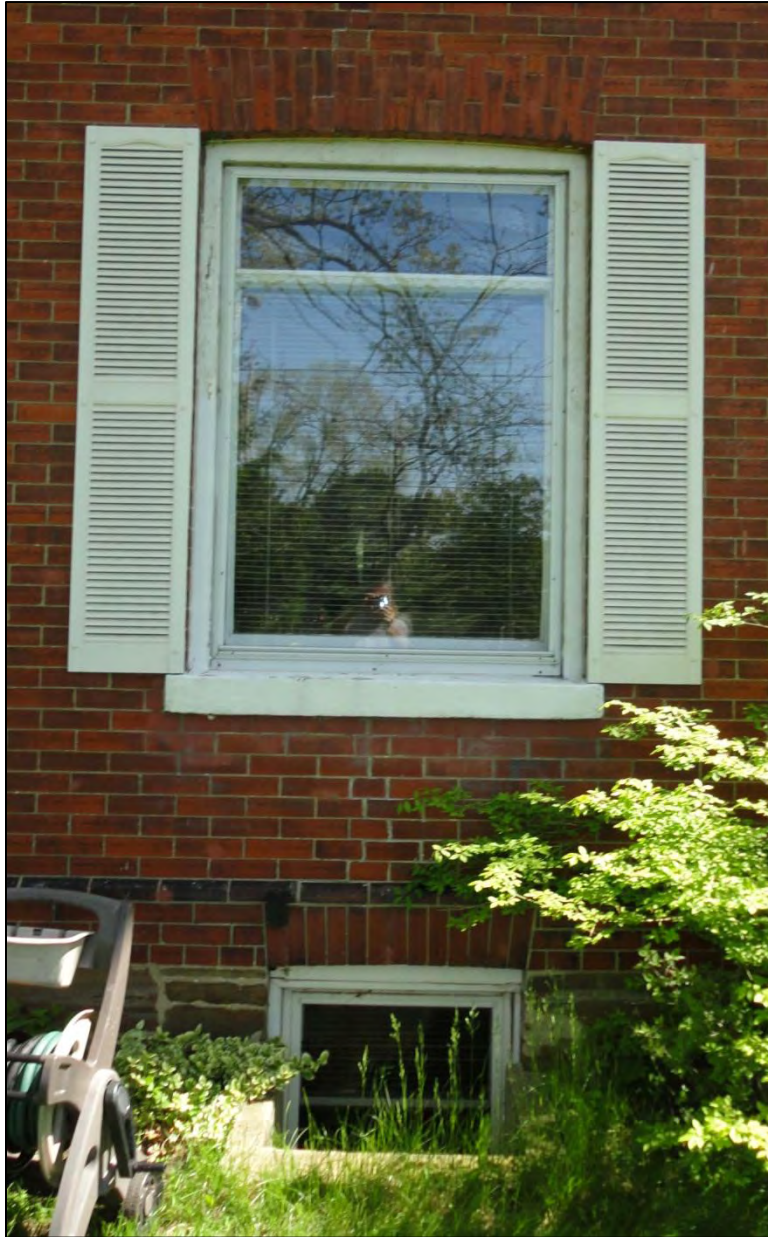
Windows, Ground Floor and Basement, West Elevation
