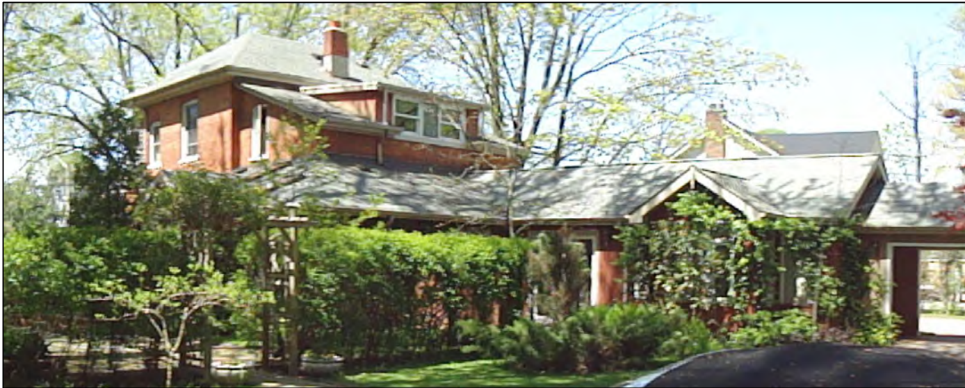
South and East Elevations
