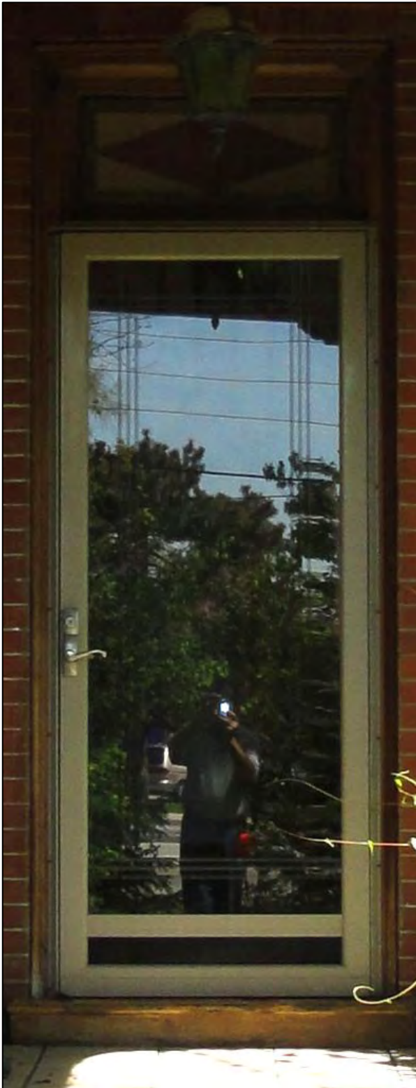
Front Door Opening – West Elevation
