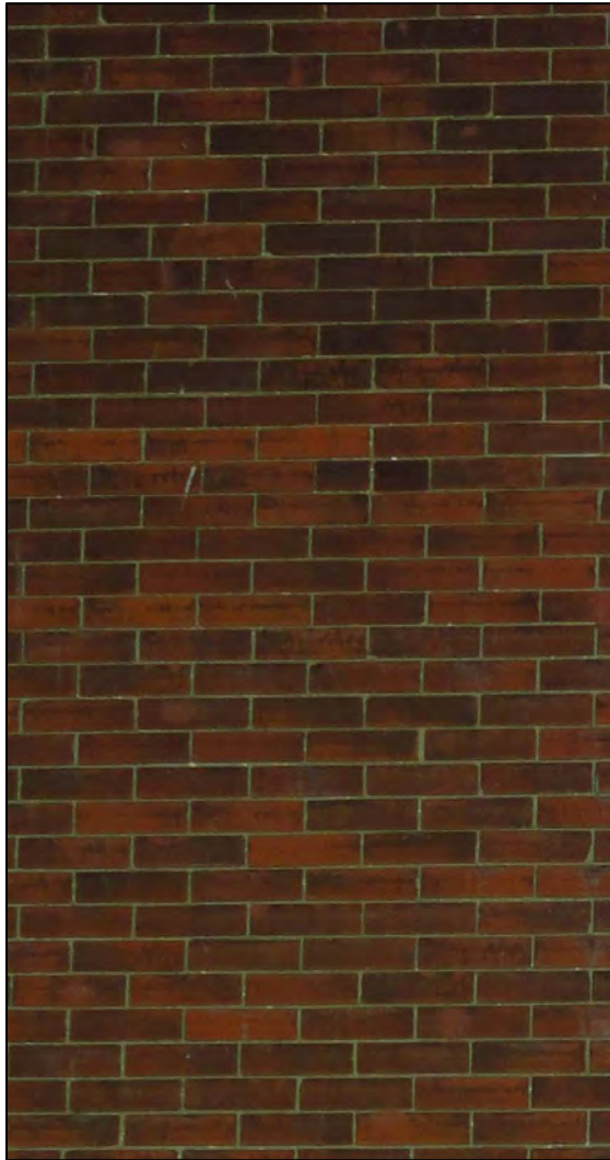
Typical Brick work, West Elevation
