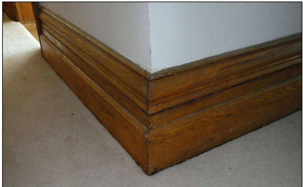
Upper Floor – Hall Basement stairs looking up to side wing Baseboard
