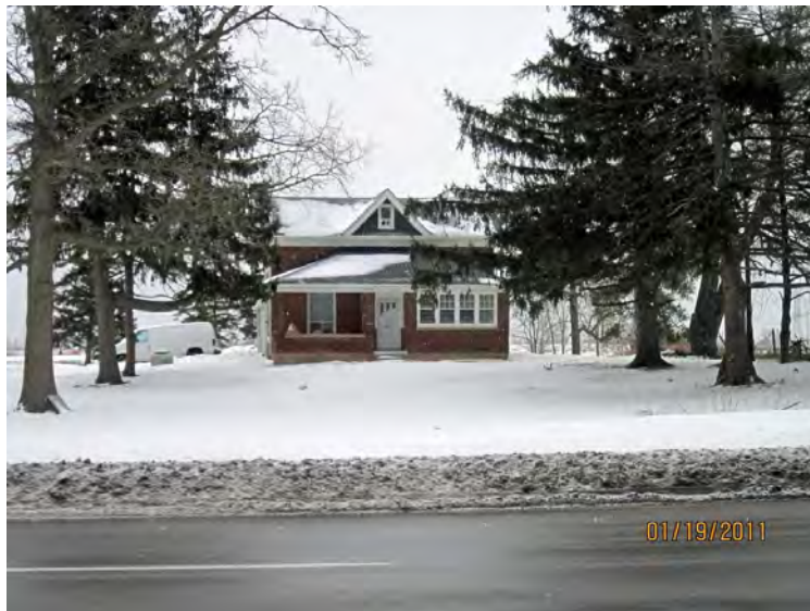
Photograph 7 Original Structure and Porch facing South
