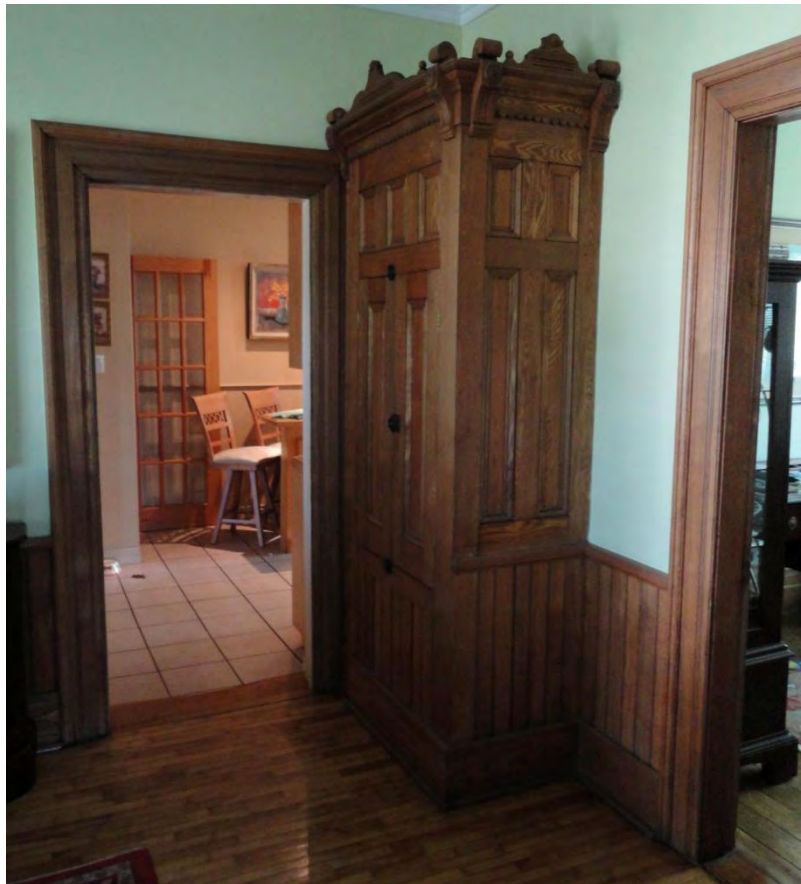
Ground Floor – North-east Room – View of Door Casings, Wainscoting & Built-in Dumbwaiter
