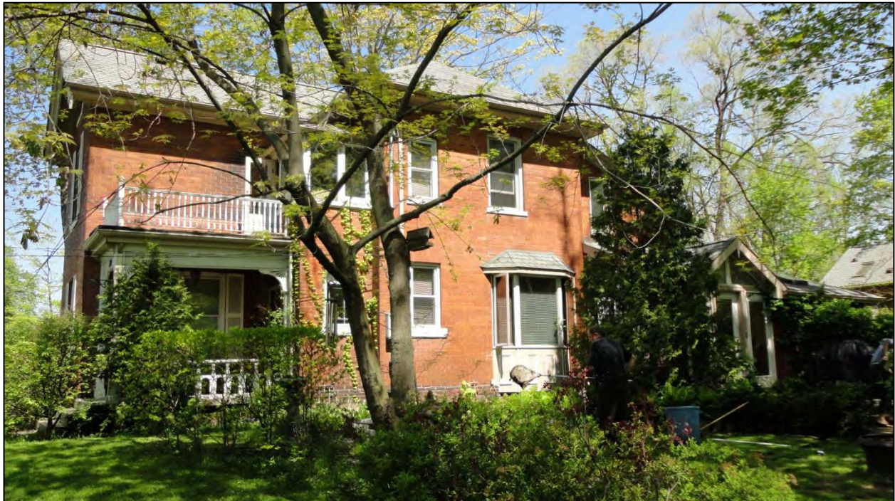
South Elevation, west end
