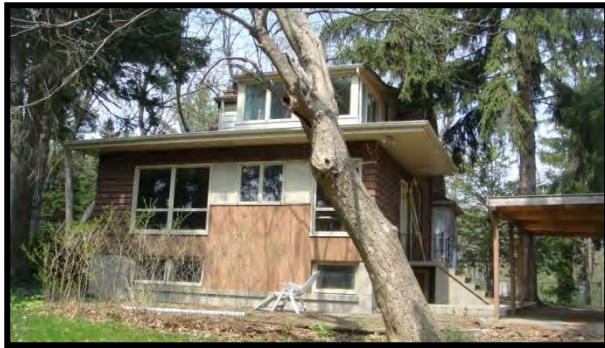
View from rear yard viewing NAS associated with the Credit River
