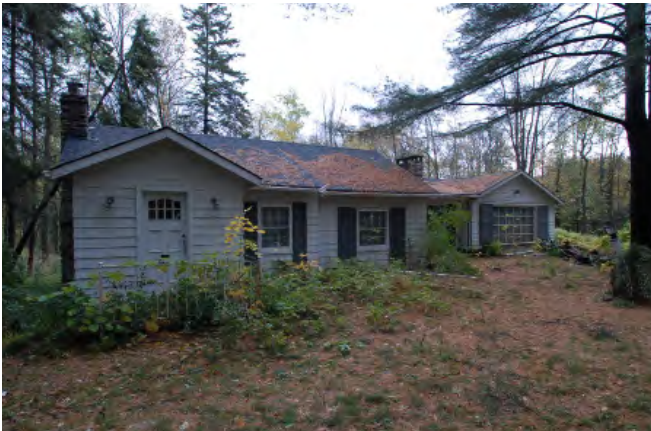
North East Corner (Original Entry)
