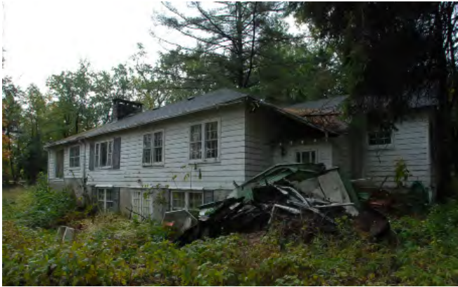
North East Corner (Basement Walkout)
