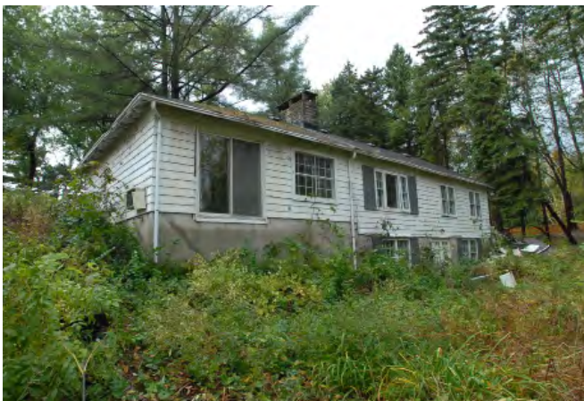
South East Corner
