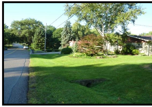
Photo 4 – View from Rear Yard looking Southwest
