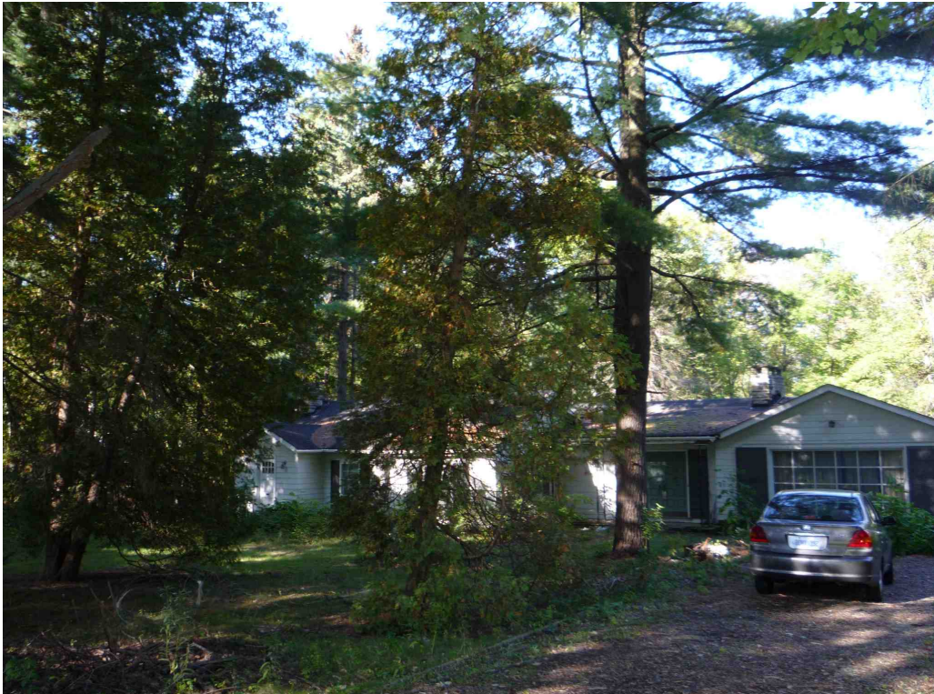
Photograph 1: View of front yard showing T100 and existing house and driveway to be demolished.
