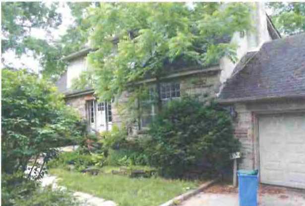
Plate 3: Looking south at two storey residence.
