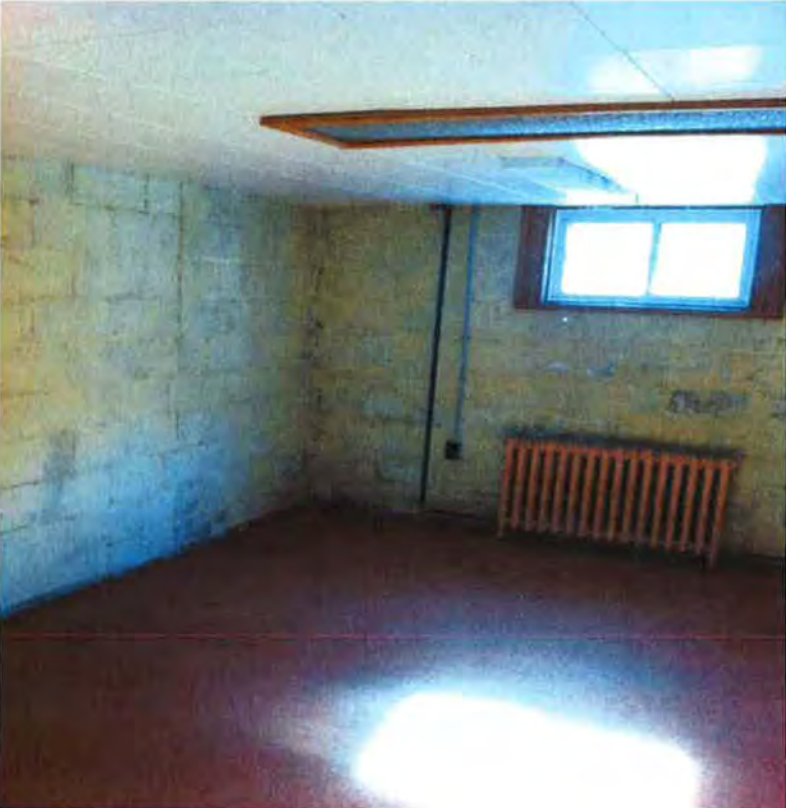
BASEMENT UNFINISHED ROOM
