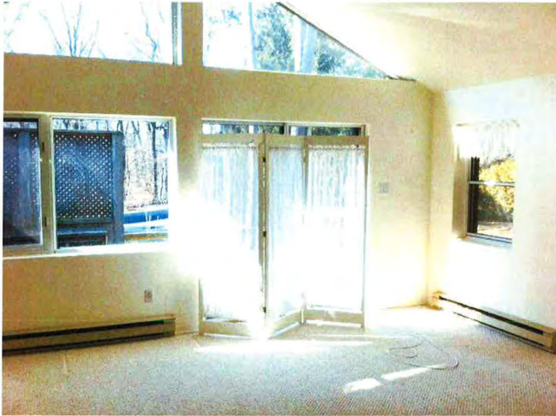
EXISTING INTERIOR VIEW
