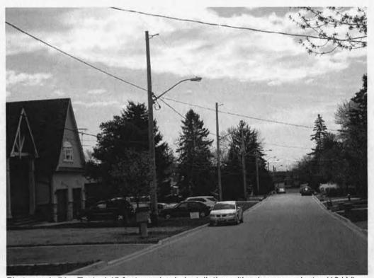
Photograph #4 - Typical 45 foot wood pole installation with primary conductor (16 kV)
