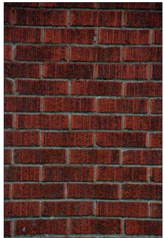
Figure 9 rug brick detail
