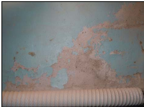
Figure 13 CIP concrete foundation wall (inside)
