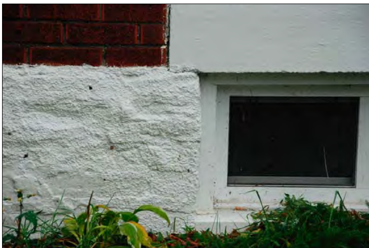
Figure 8 parged & painted concrete foundation, lintel & sill
