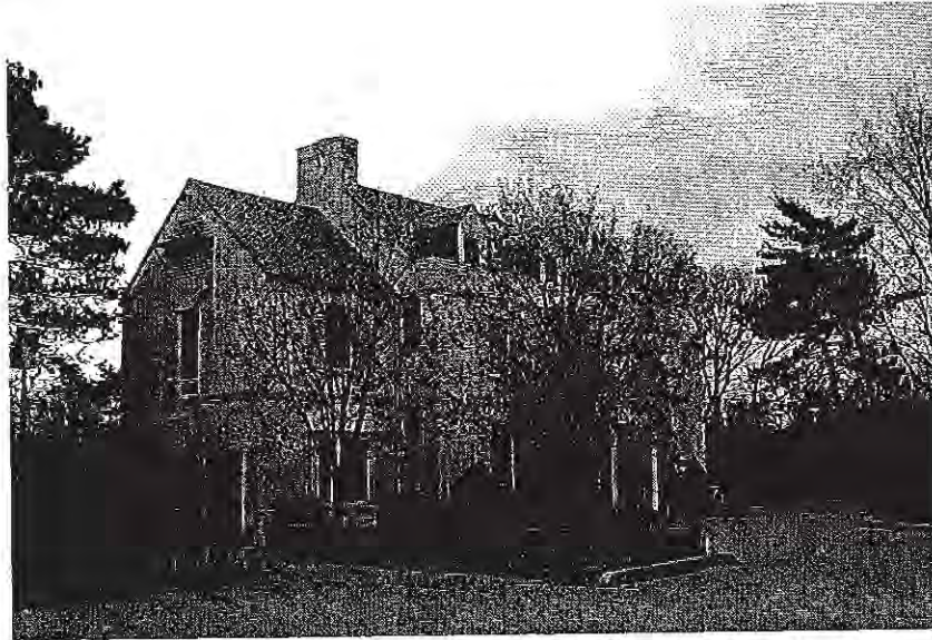
Figure 9: Bell Gairdner Estate, April 2006. View facing southwest.
