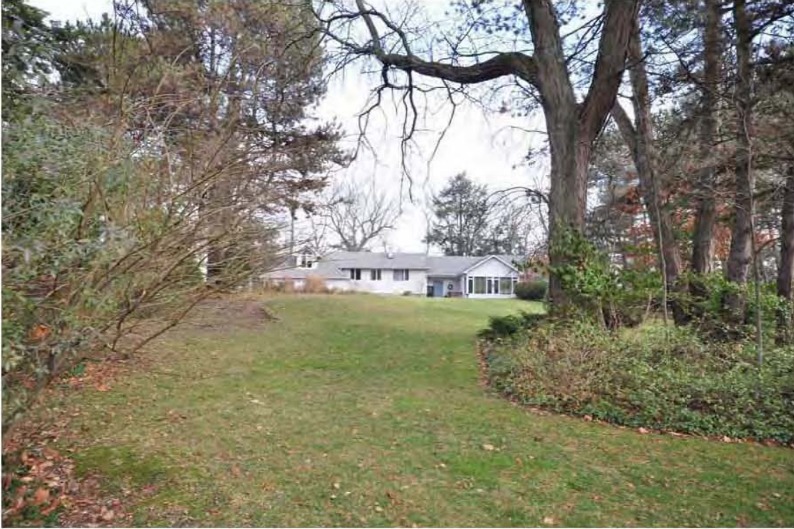
Front Elevation –view from street (west elevation)
