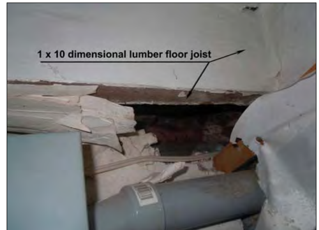
Figure 14 floor /ceiling joist
