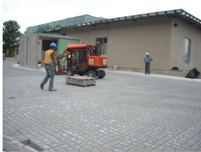
Construction of Station 106
