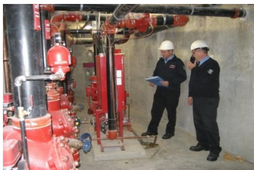
Fire Safety Inspection
