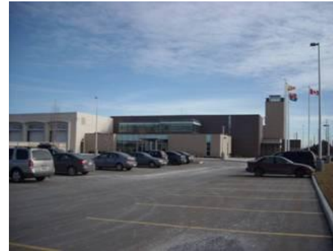
Fire Station 116 and Peel Regional Paramedic Reporting Station
