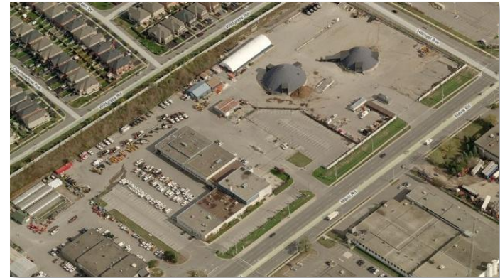
Arial view of the Mavis Public Works Facility at 3185 Mavis Road. The Administrative Building will undergo renovations to accommodate the New Traffic Management Centre.
