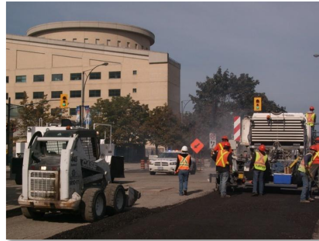
Work crews rehabilitating Duke of York Boulevard
