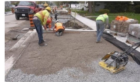
Construction workers completing the LID Project in the Lakeview Area
