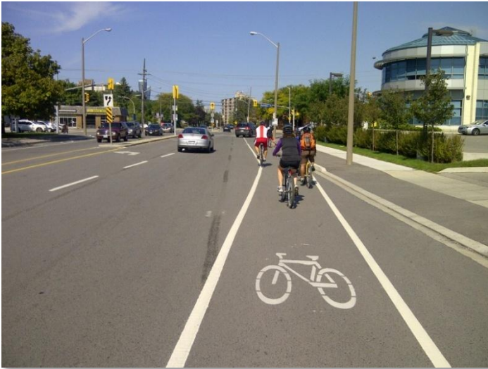
New cycling facility along Camilla Road
