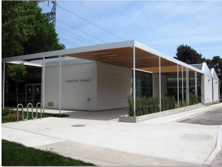
Lakeview ISF renovation location
