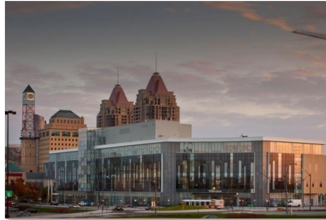
Sheridan College Phase I, Hazel McCallion Campus. Looking ahead to open Phase II.
