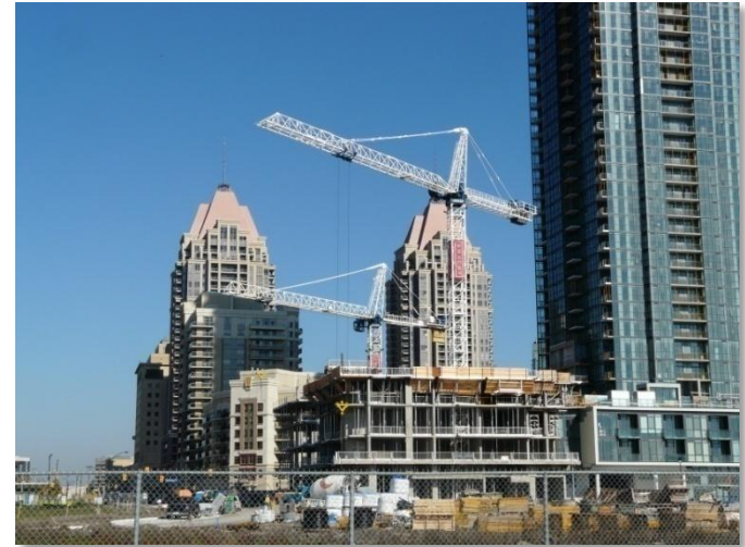
Residential high density development under construction in the city core.
