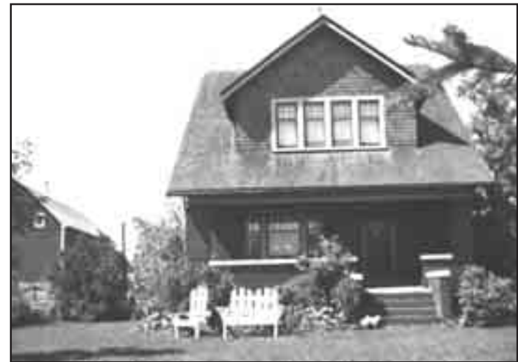
▲ McCracken House and Barn
