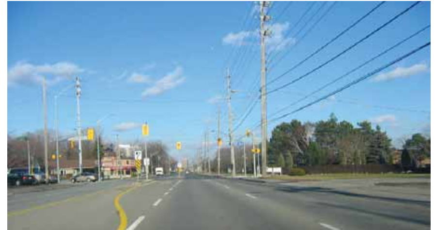
Lakeshore Road is four lanes wide with a continuous centre turning lane.
