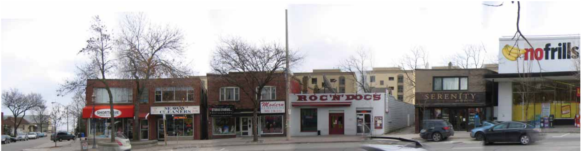
Existing commercial built form on south side of Lakeshore Road.
