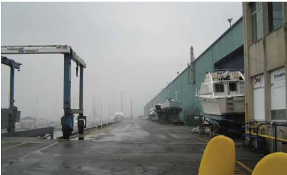
View of marina (and fog) looking towards Lake Ontario on east side of marina building.
