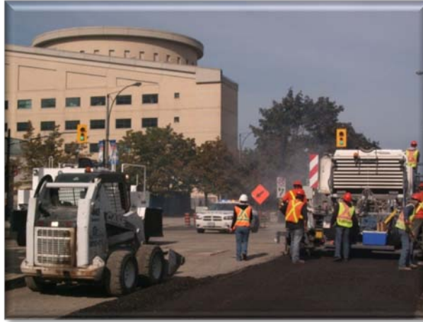
2010 Duke of York Road resurfacing improvements
