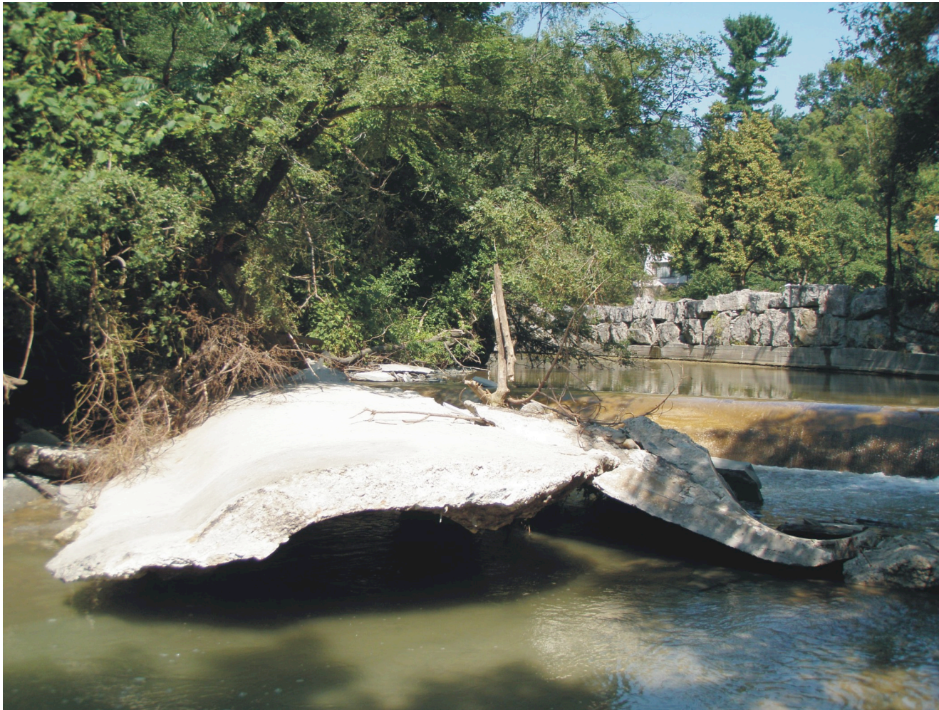
Figure 2 Municipal Infrastructure Damages - Dislodged Sanitary Sewer Cap
