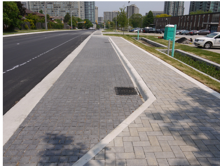
Low impact development features along Elm Drive West
