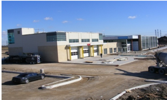
Garry W. Morden Centre Administration Building
