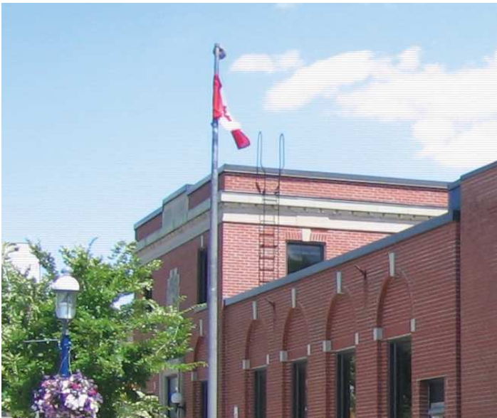
Figure 5.2 - Brick and limestone masonry to be salvaged from upper 2nd Floor
