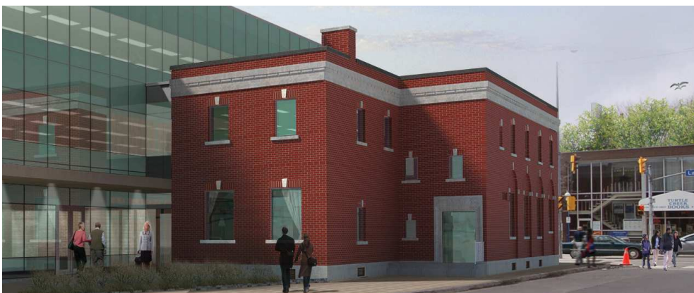
Figure 6.2 - South and East rebuilt walls to match existing 1931 window openings and masonry details
