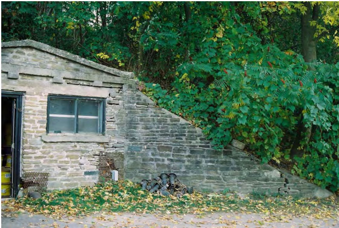
Fig. 23 Another view of former pump house, showing the western flanking buttress
