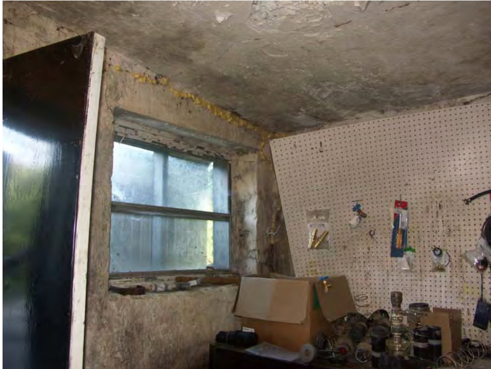
Fig. 25 Interior view of former pump house, showing poured concrete construction
