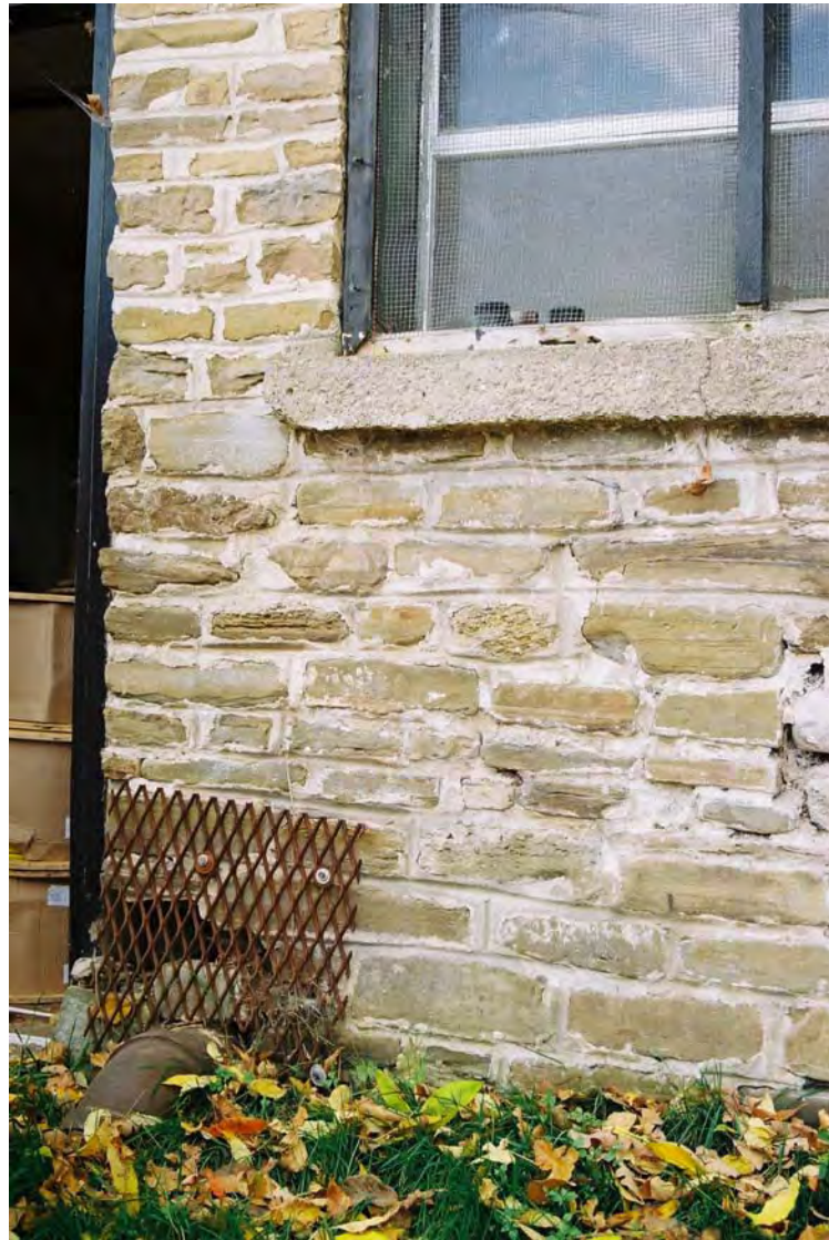
Fig. 24 Detail of rough-hewn Credit Valley sandstone face on former pump house, its concrete window sill and cast-iron intake pipe at ground
