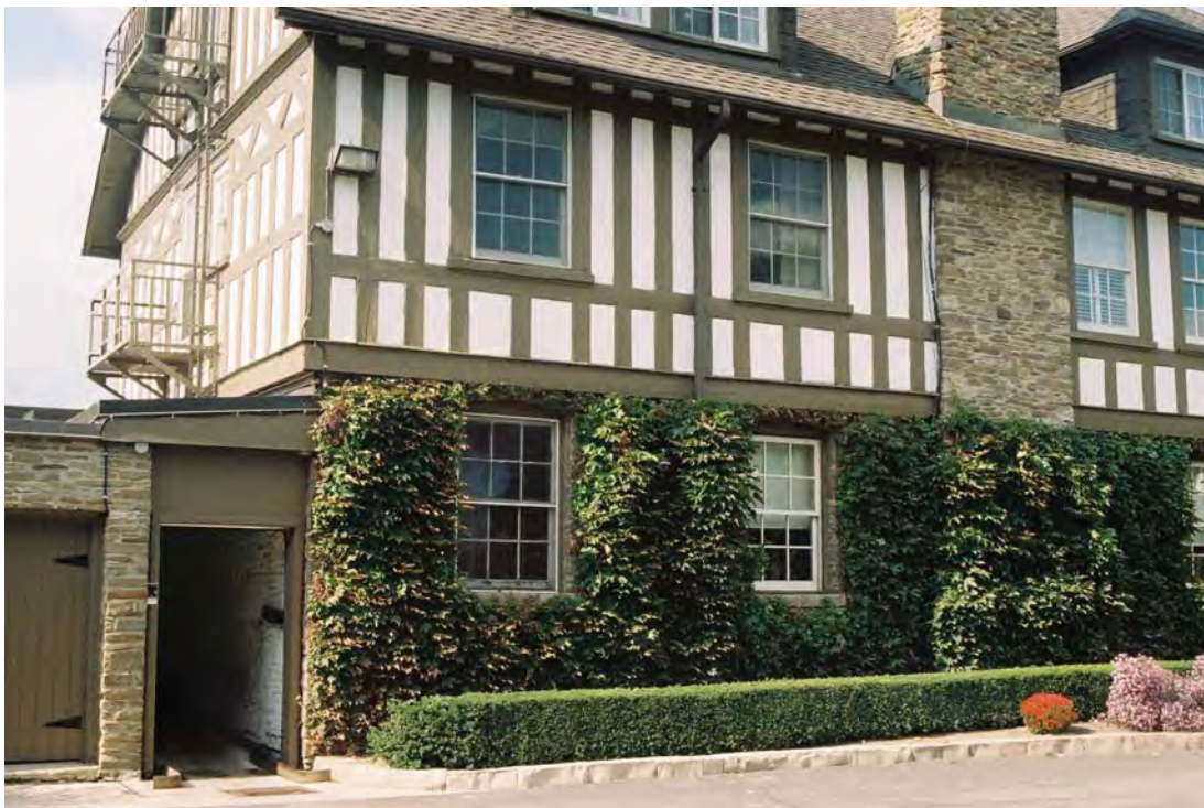
Fig. 17 Detail of clubhouse, showing rough-hewn Credit Valley sandstone ground floor and chimney and upper walls in mock half timbering
