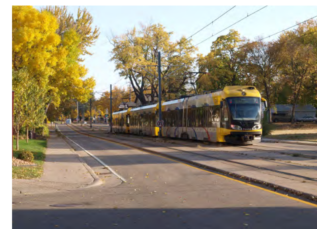
Centre-pole catenary system in Minneapolis (centre-running with one traffic lane on each side)
