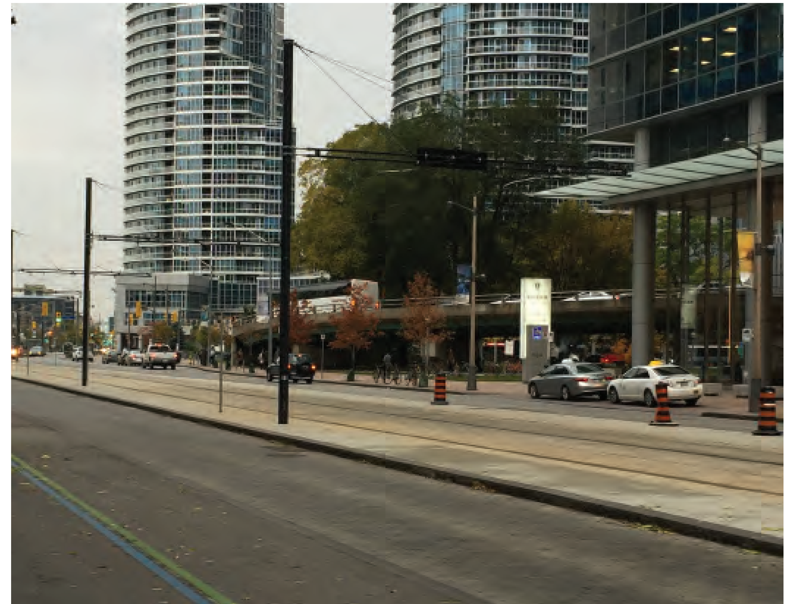
OCS poles on Queen's Quay in Toronto
