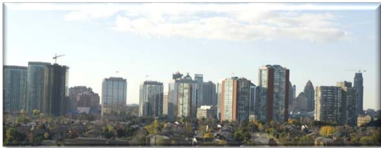
Existing apartment buildings and construction of apartment units in the downtown
