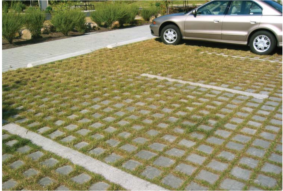
Green paving solution for parking.
