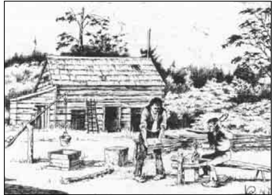
▲ Building a Cabin (Frederick R. Bercham)
