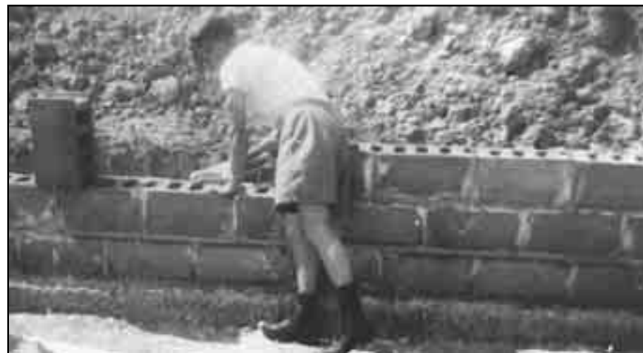
▲ George Dyer laying the foundation for his house (Photos courtesy of Mr. and Mrs. Ron Dyer)
