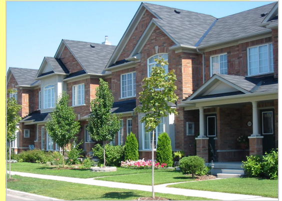
Continuous sidewalks, street trees, year-round landscaping, and porches enhance the appearance and safety of the street
