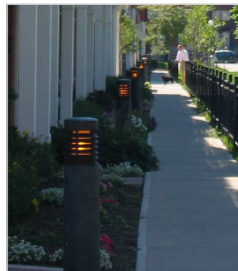
Bollard lighting to illuminate a pedestrian path
