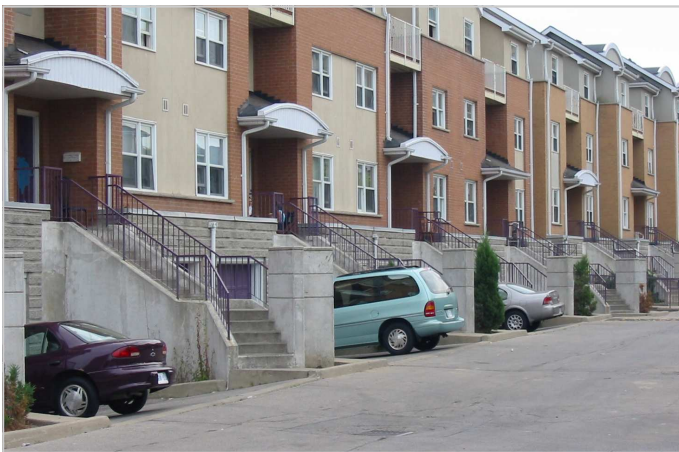
Avoid basement garages with sloped driveways next to the street
