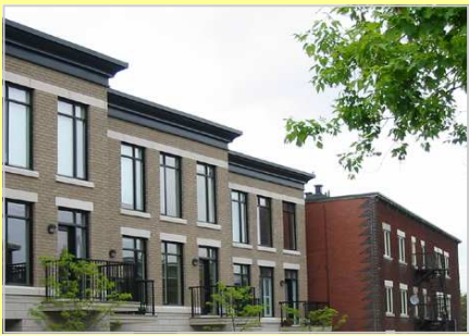
Continuing the lines and rhythm of neighbouring façades gives coherence to the streetwall
