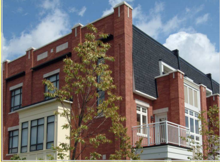
Rooflines characteristic of surrounding development provide continuity and reinforce neighbourhood identity
