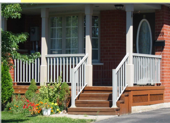
A porch feature is more functional when generous in width and depth
