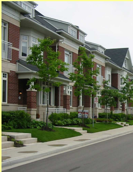
Landscaping and a well-defined building edge enhance the streetscape
