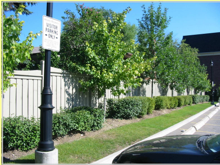
A 3 metre wide (10 feet) landscape area with decorative fence separates parking area from adjacent yard
