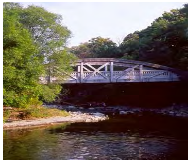
Figure 8-14: The Middle Road Bridge, located at the end of Sherway Drive at the Etobicoke Creek, is an engineering wonder. Built in 1909, it is the first concrete bow bridge of its kind in Canada.
