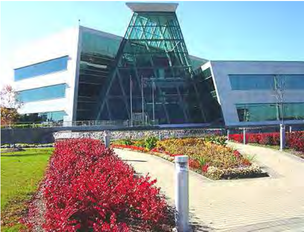
Figure 8-28: Architecturally expressed entrance features and defined landscaping, provide a welcoming gesture and denote the sense of principal access to the building. (Biovail Pharmaceutical Corporation, Meadowvale Business Park)
