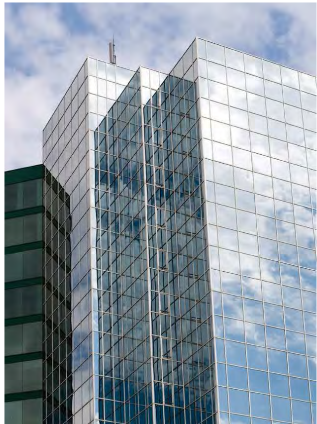
Figure 9-4: Over the years Mississauga has been able to attract many diverse businesses. Many of these offices have concentrated in the city's Corporate Centres, Employment Areas and Downtown. In the future, the City will promote increased office use and activity within the Downtown.
