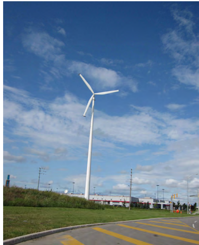
Figure 9-11: A 31 m wind turbine unveiled at the Lisgar GO Station in April 2009 generates as much as 80 per cent of the station's power. The site, located at Tenth Line and Argentia Road, was chosen for the wind turbine because of heavy prevailing winds from the west and its open fields.
