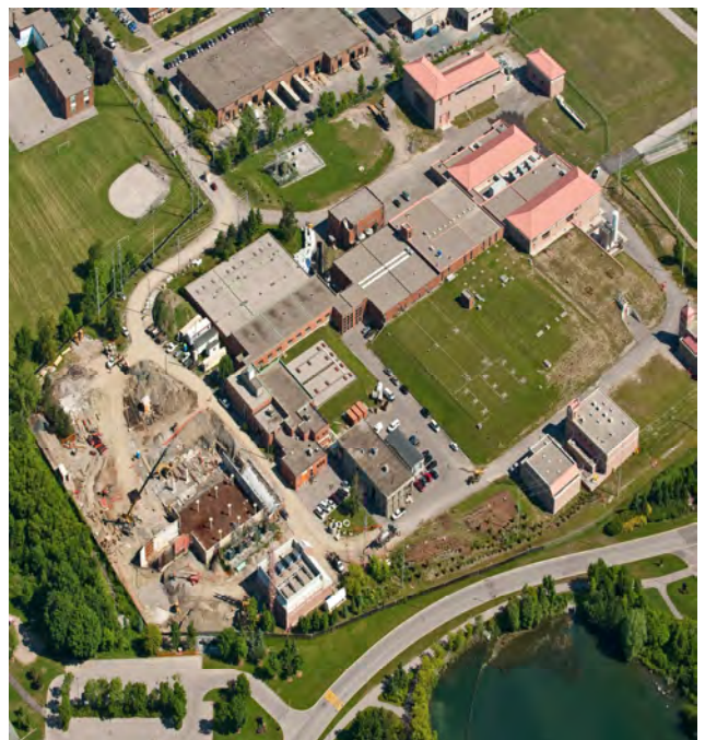
Figure 9-8: The G. E. Booth Wastewater Treatment Facility is located on the shore of Lake Ontario in Mississauga and is operated by the Region. This plant processes the wastewater from homes and businesses in Bolton, Caledon East, Brampton and the eastern parts of Mississauga. Three trunk sewers lead to the Lakeview plant with the total daily capacity of 448,000 cubic meters of wastewater.
