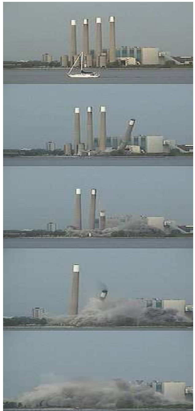
Figure 19-6: The Lakeview Generating Station, also known as the Four Sisters, ceased operations in April 2005 after 43 years and was demolished in June 2006. The former coal burning station had been in operation since the early 1960's.
