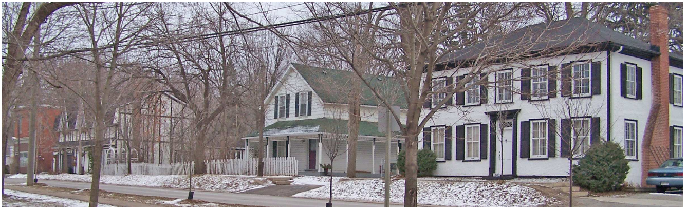
Figure 7-7: Heritage Conservation Districts enable the City to manage and guide change through the adoption of a plan and guideline for the conservation, protection and enhancement of each area’s special character. Meadowvale Village, at Old Derry and Second Line roads, is a historic community within the modern City of Mississauga. The City recognized the significance of Meadowvale Village in 1980 by designating it a Heritage Conservation District pursuant to the Ontario Heritage Act , the first designated in Ontario. More recently, Port Credit Village was designated a Heritage Conservation District in 2004.
