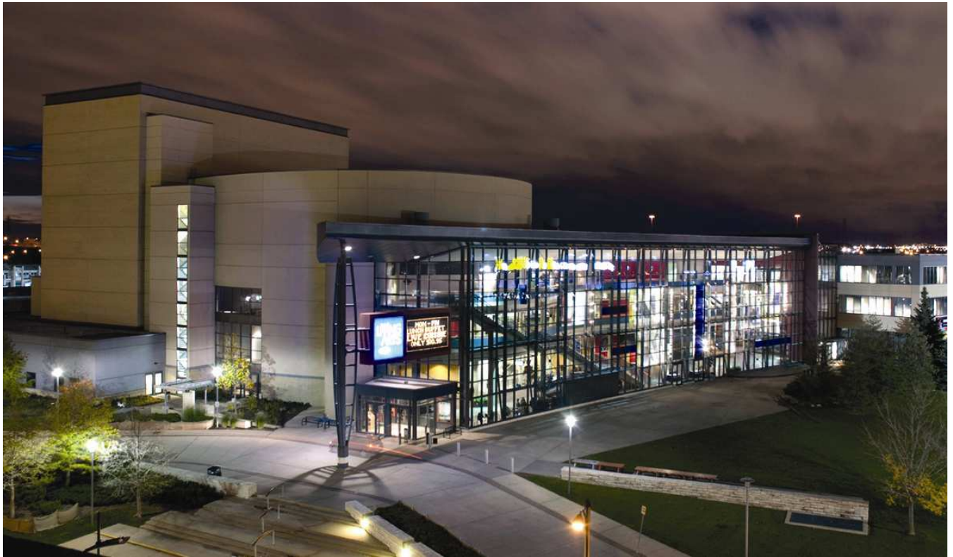
Figure 7-9: The Living Arts Centre (LAC) opened its doors on October 7, 1997, adding an exciting cultural dimension to Mississauga's Downtown. Serving as an important resource for the arts, education and business, LAC features over 225,000 square feet of multiple performance venues, studio spaces and exhibition display areas. The LAC is a valued cultural resource that benefits the community.
