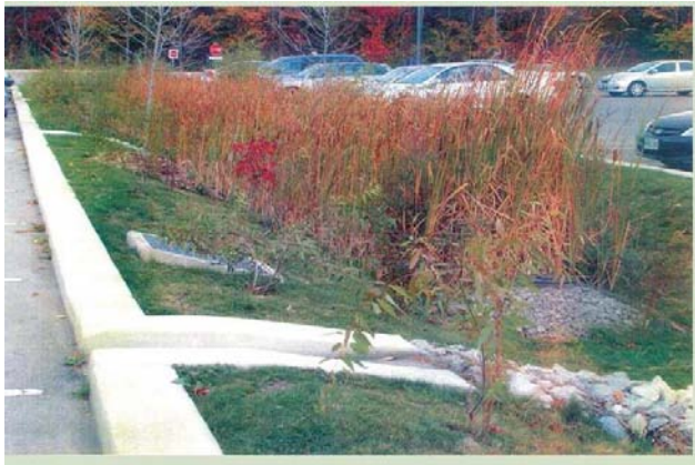
Figure 9-34: Bioretention features, such as stormwater best management practices , are encouraged to be incorporated in site development.
