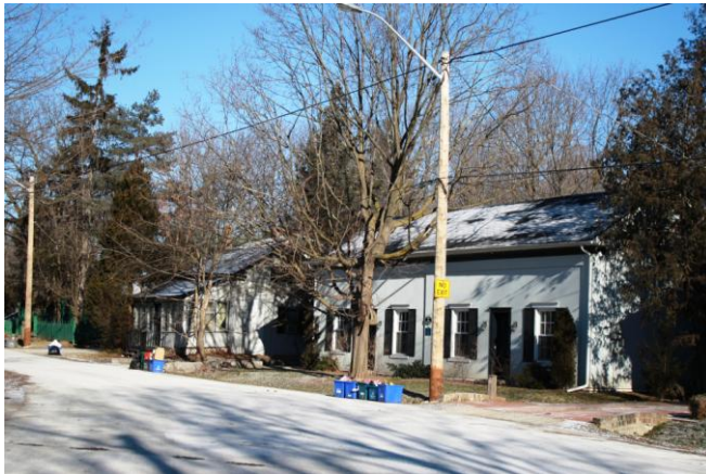
These original houses have the ground floor at grade, (photo 2013)
