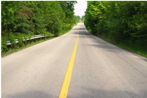
Second Line west looking north, 2012
