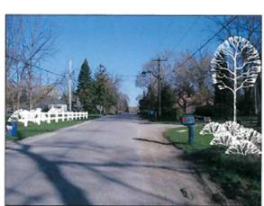
Figure 10. The rural road cross section consists of highly textured pavement (tar and chip) gravel shoulders and turf boulevards. Fencing or shrub borders may be added to define the edge of the front yard.
