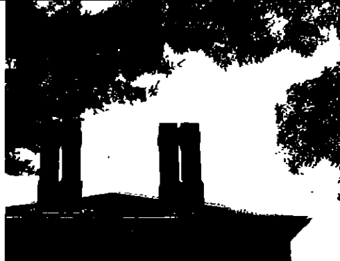
Chimneys on the northwest side of the house.
