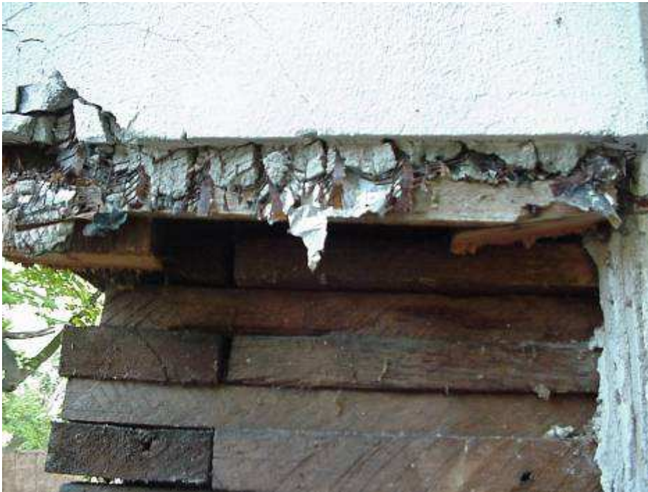
Detail of corner, stacked plank construction.
