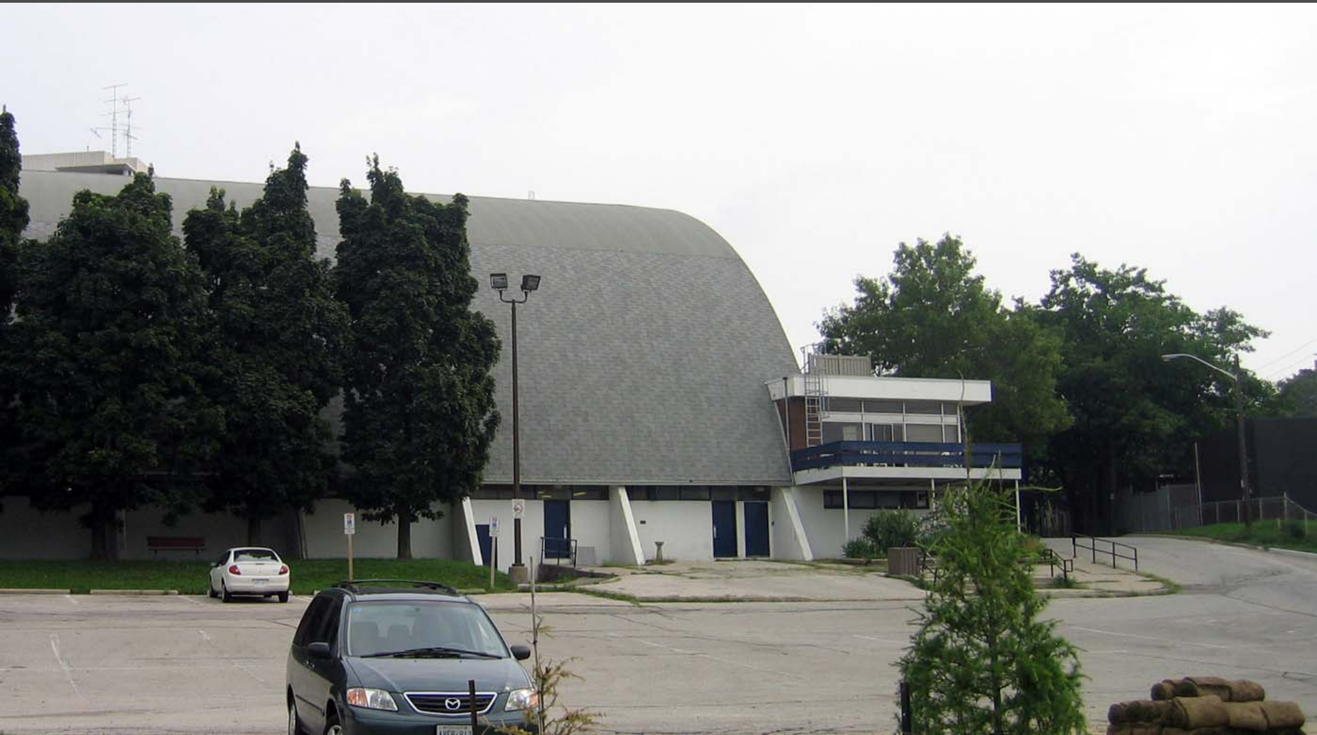
Existing View from the Parking Lot
