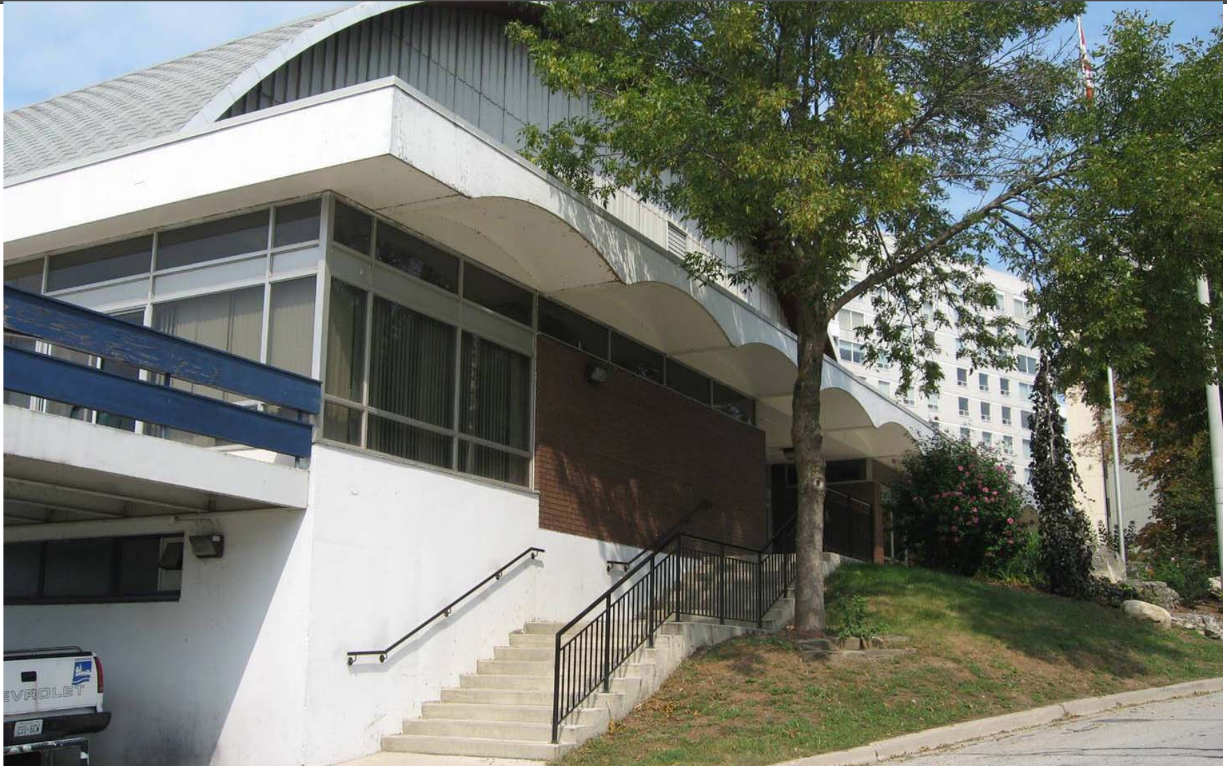
Existing View from Driveway
