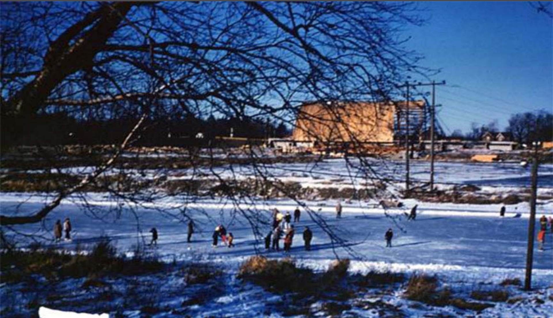
Old View from Lakeshore Road during construction (1959)
