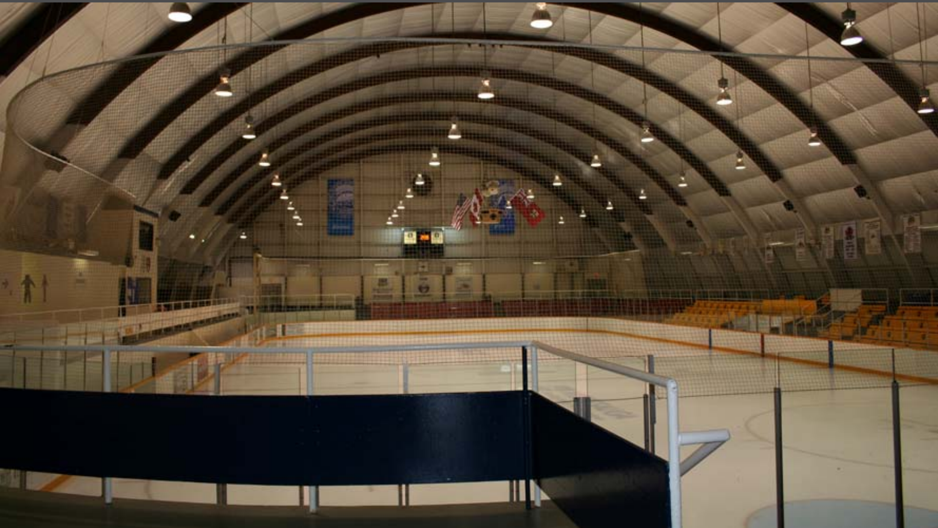
Existing View from Upper Entrance into the Arena
