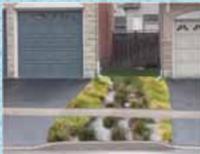
Construction of bioretention facility could store up to half of the runoff for the August 2009 storm
