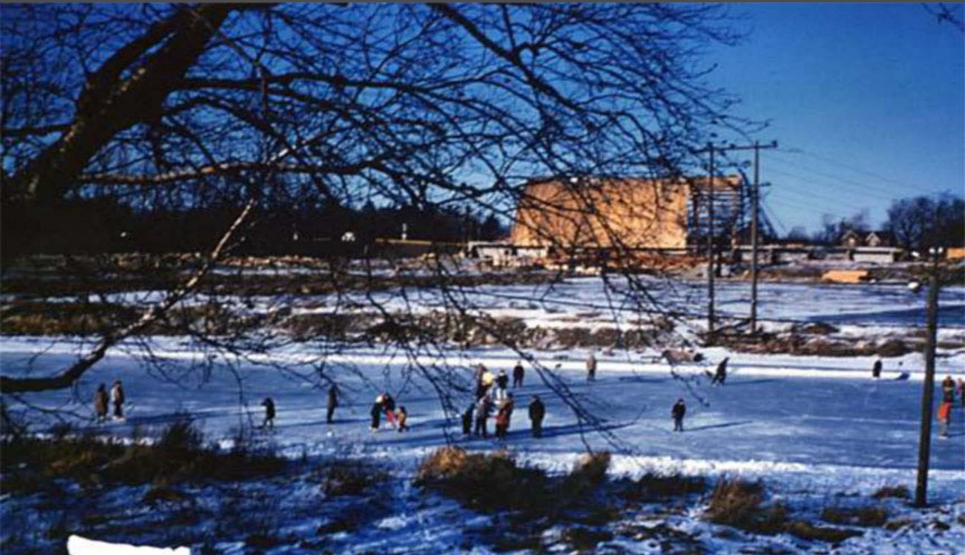
View from Lakeshore Road during Arena construction (1959)
