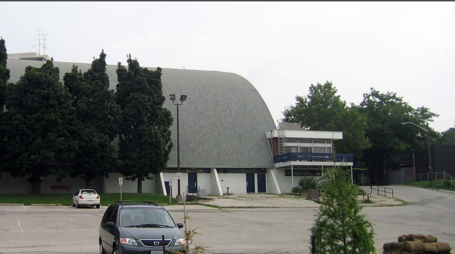
Existing View from the Parking Lot
