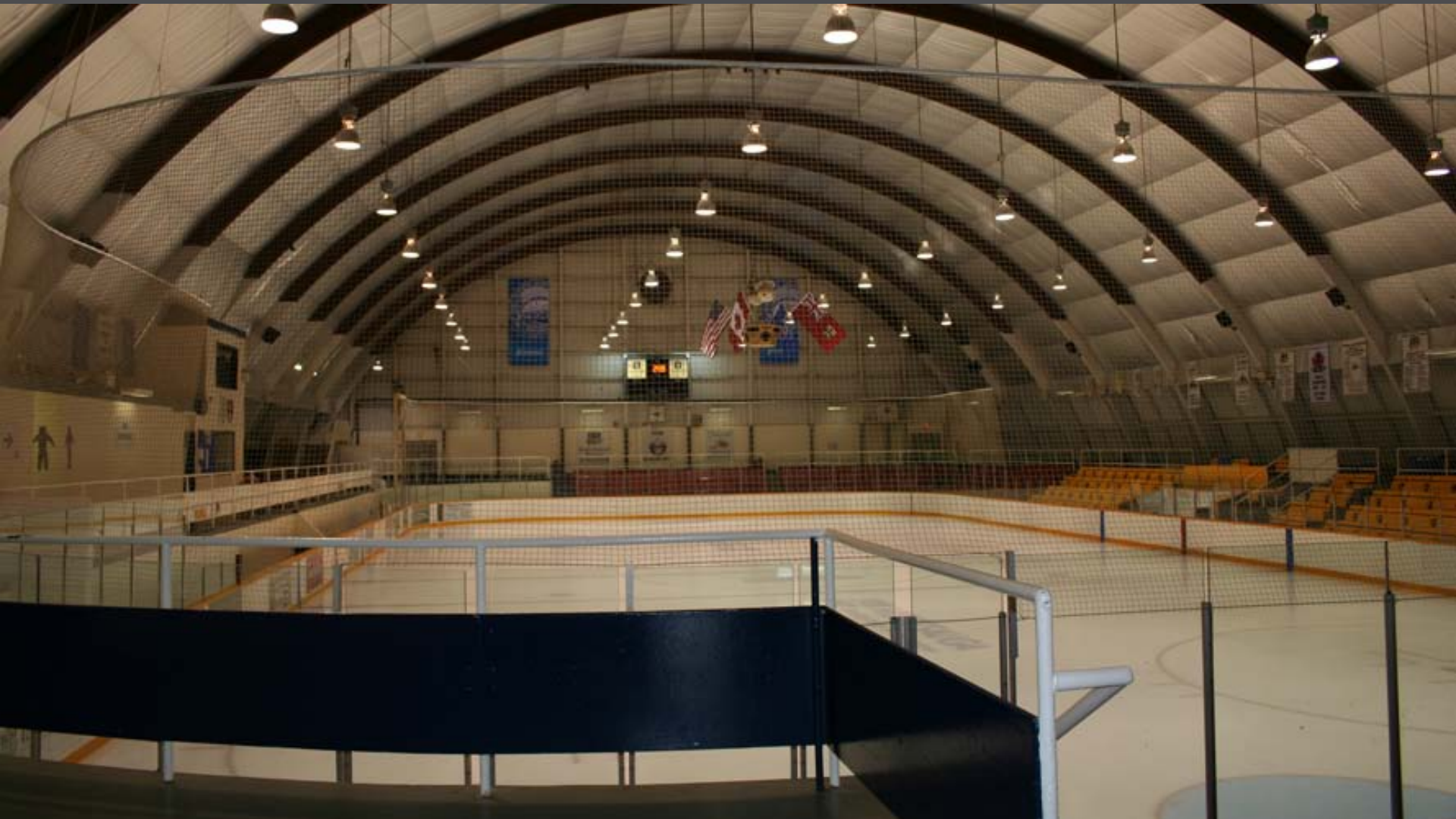
Existing View from Concourse into the Arena
