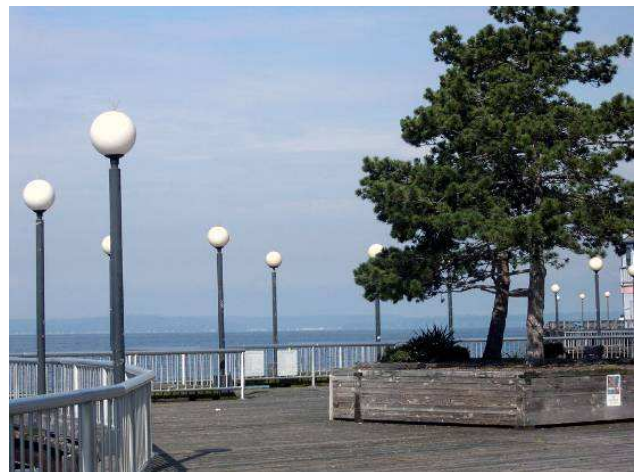
Pedestrian scale lighting provides illumination for public amenity areas, sidewalks and pathways, as illustrated above.
