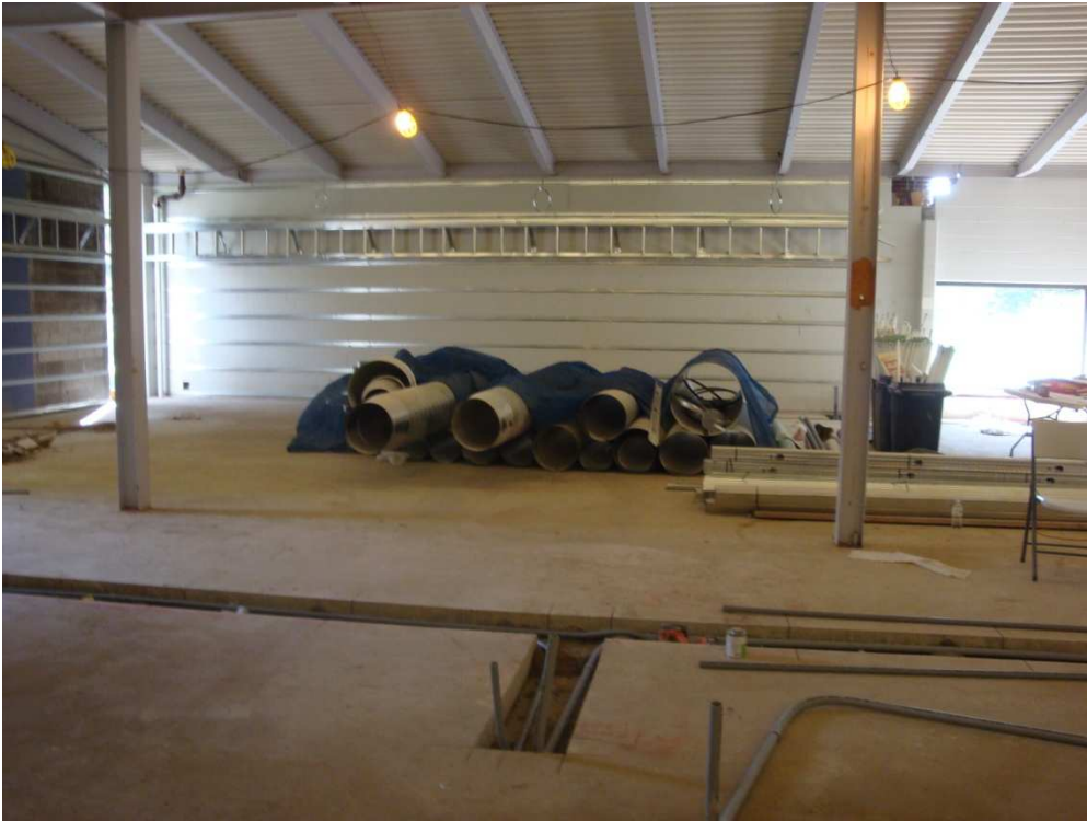
South Interior Wall
