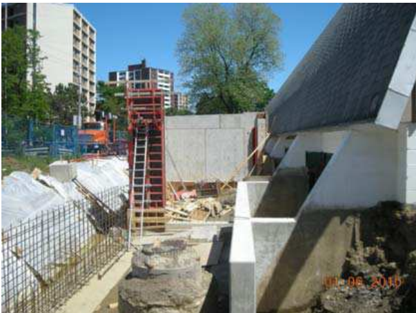
Foundation of new storage room
