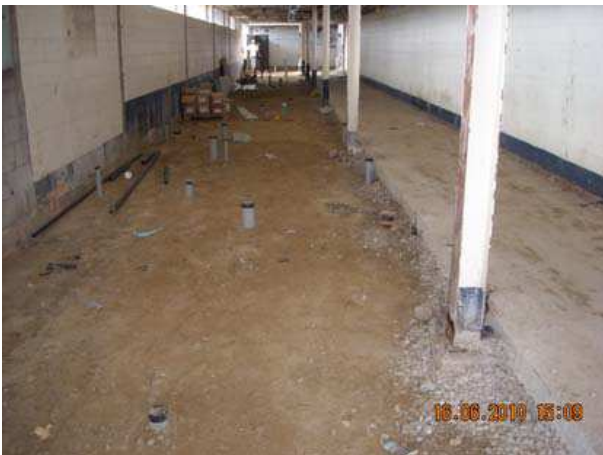
Underground plumbing work
