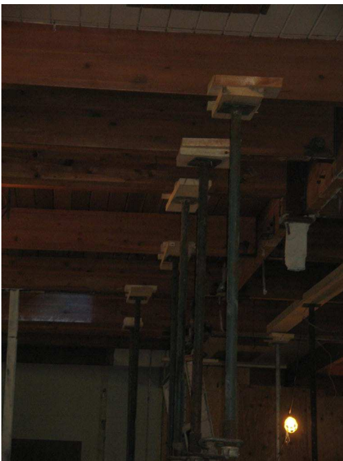
Shoring up the ceiling
