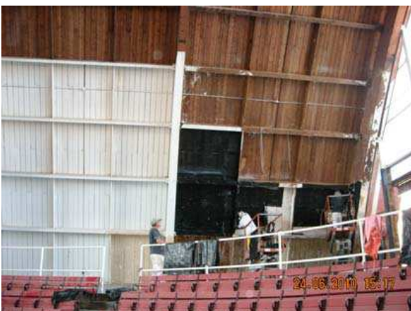
Paint removal work ongoing
