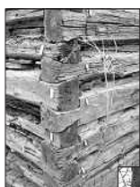
Prior to dismantling, all the logs were numbered and tagged.
