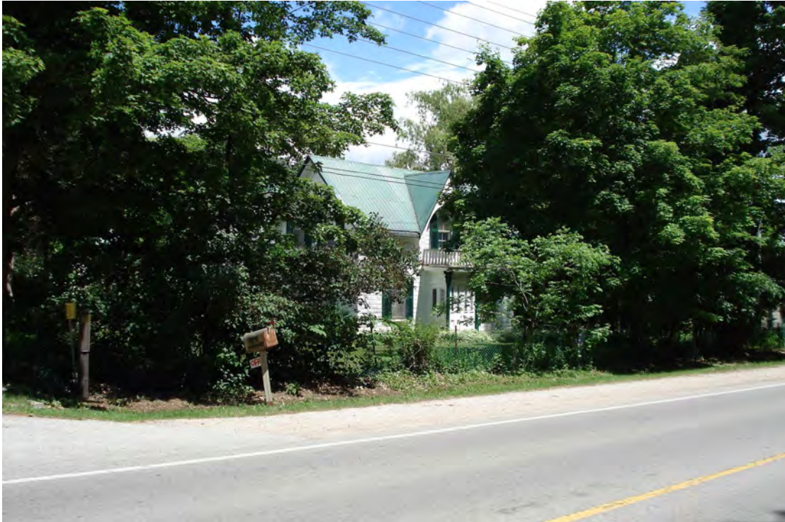
Figure 12: West face, June 2008.
