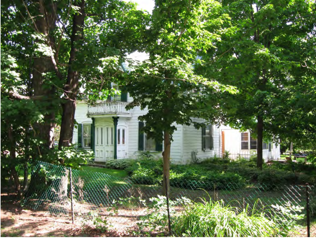
Figure 14: Southwest view, August 2009.
