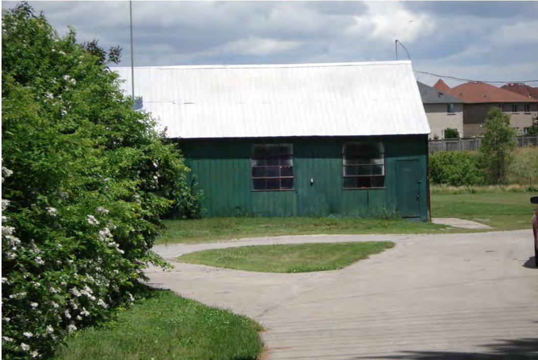
Figure 16: West face of large outbuilding, June 2008.
