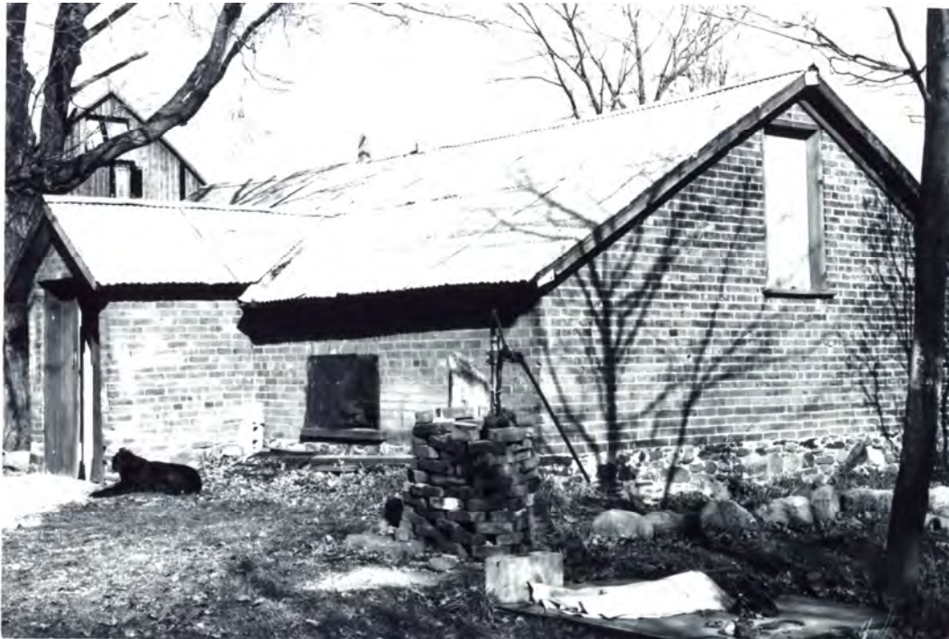
Figure 9: Small Outbuilding, December 1976.
