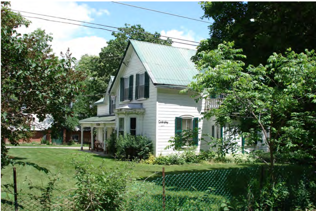
Figure 13: Northwest view, June 2008.
