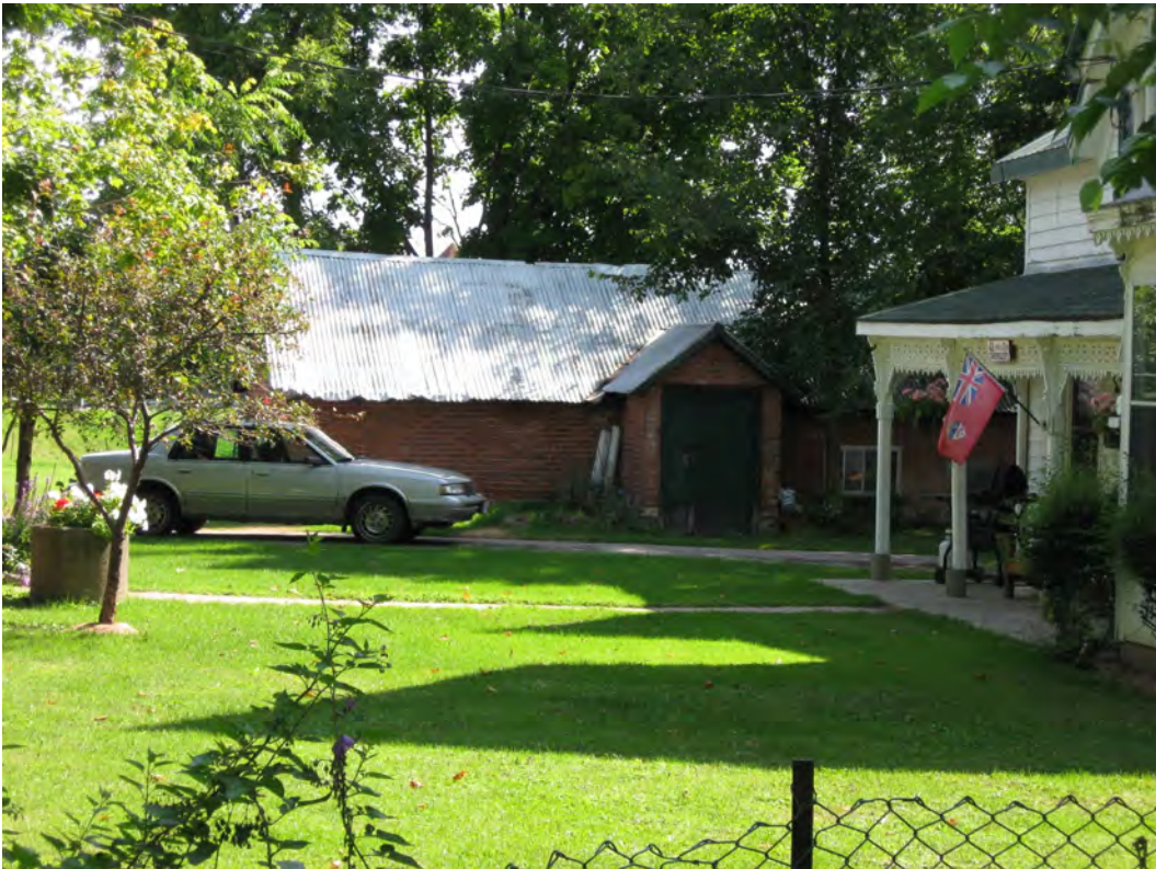
Figure 15: West face of small outbuilding and north side of house, August 2009.
